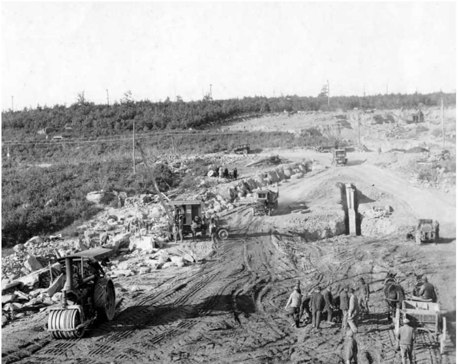
Mules and steam engines provided much of the brawn needed to build the Wallenpaupack dam, as seen in this view of the earthen north embankment of the dam.
