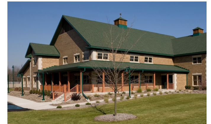
PARCC-Side Clean Water Plant, Plainfield Charter Township
