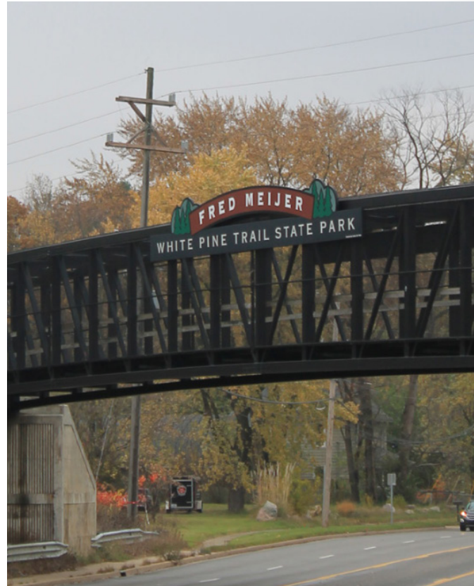
White Pine Trail West River Dr Overpass, Plainfield Charter Township
