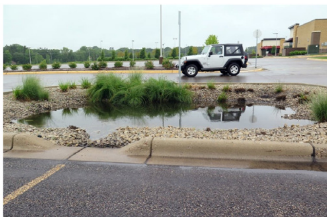
A rain garden at the Argenta Hills development collects rainwater from the Target parking lot. Rather than constructing stormwater ponds and a series of pipes and pumps to carry the water away from the site, engineers used green infrastructure and low-lying basins to create a system that can handle even the largest storms. ■ Elizabeth Dunbar | MPR News
