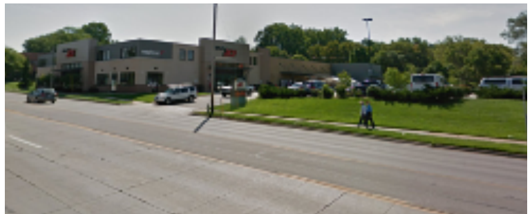
Sidewalks and limited driveways make pedestrian travel safer.
