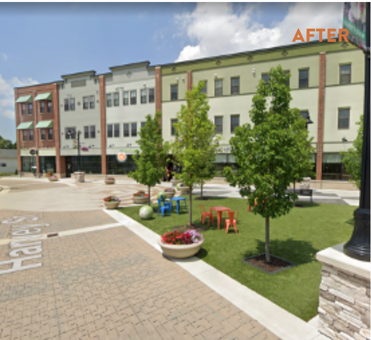
Harvey Street in Hudsonville
