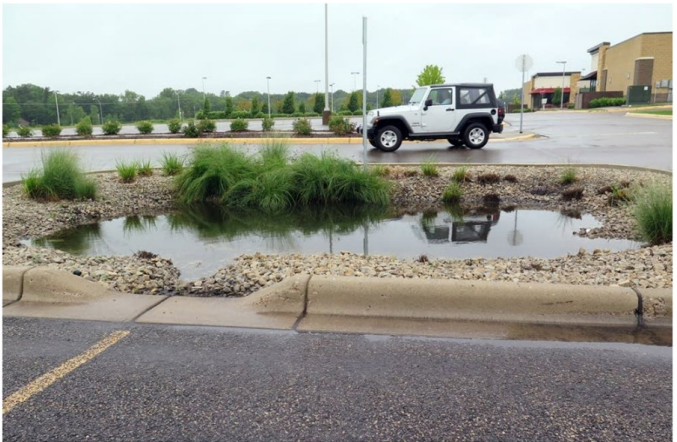
A rain garden at the Argenta Hills development collects rainwater from the Target parking lot. Rather than constructing stormwater ponds and a series of pipes and pumps to carry the water away from the site, engineers used green infrastructure and low-lying basins to create a system that can handle even the largest storms. ■ Elizabeth Dunbar | MPR News
