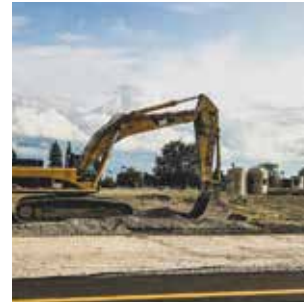
Construction Staging Sites
