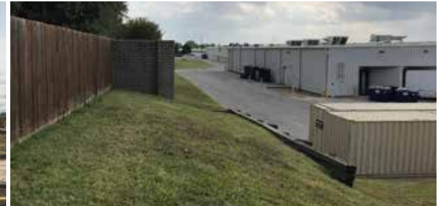
Large Outdoor Storage Areas
