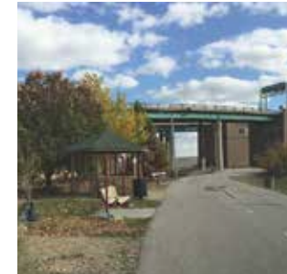
Trail under I-635 to/from KC Current soccer area
