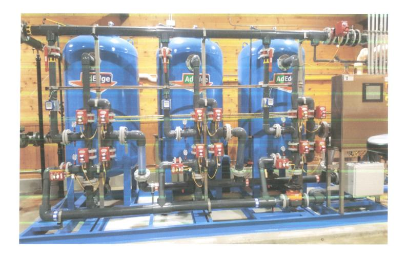
Work on the \$500,000 Junction Road Arsenic Treatment System started in March 2018 and was put in service in August. The improvements included the Arsenic Treatment System, installation of a backwash tank and two backwash lagoons, and upgrades to the electrical and SCADA systems. The fully automated system allows the District to run the system at night without oversight from District personnel.
