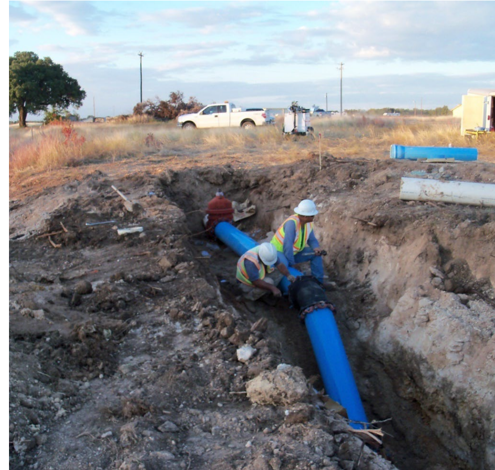
REPRESENTATIVE IMAGE OF LAYING A WATER LINE
