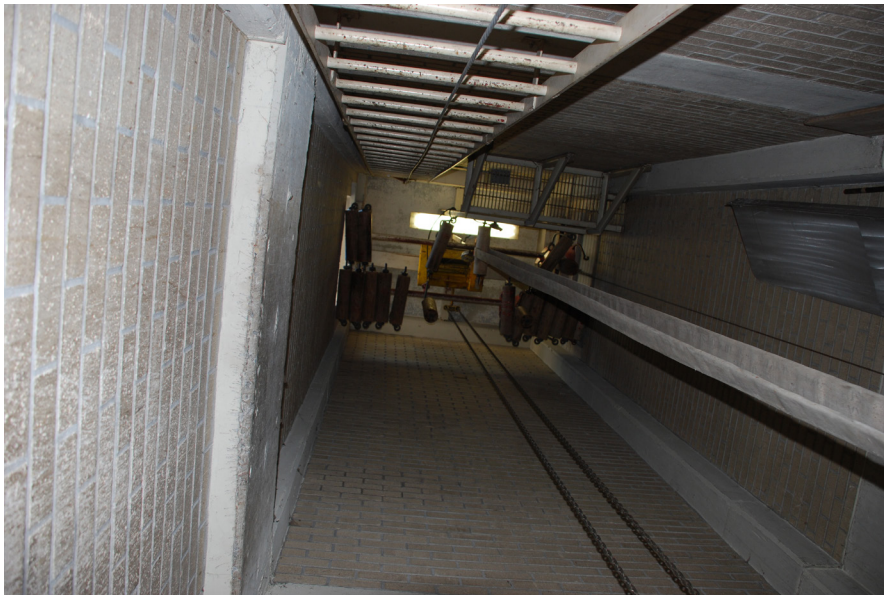
Station 1 has a "25' hose tower that was designed to allow the hanging of 50' sections of hose draped over spindles at the top of the tower. In the photo above can be seen one section of hose. The hose tower is getting little use of late because Shawnee has moved away from "cotton jacketed" attack hose. Cotton jacketed hose had to be dried before being placed back on
