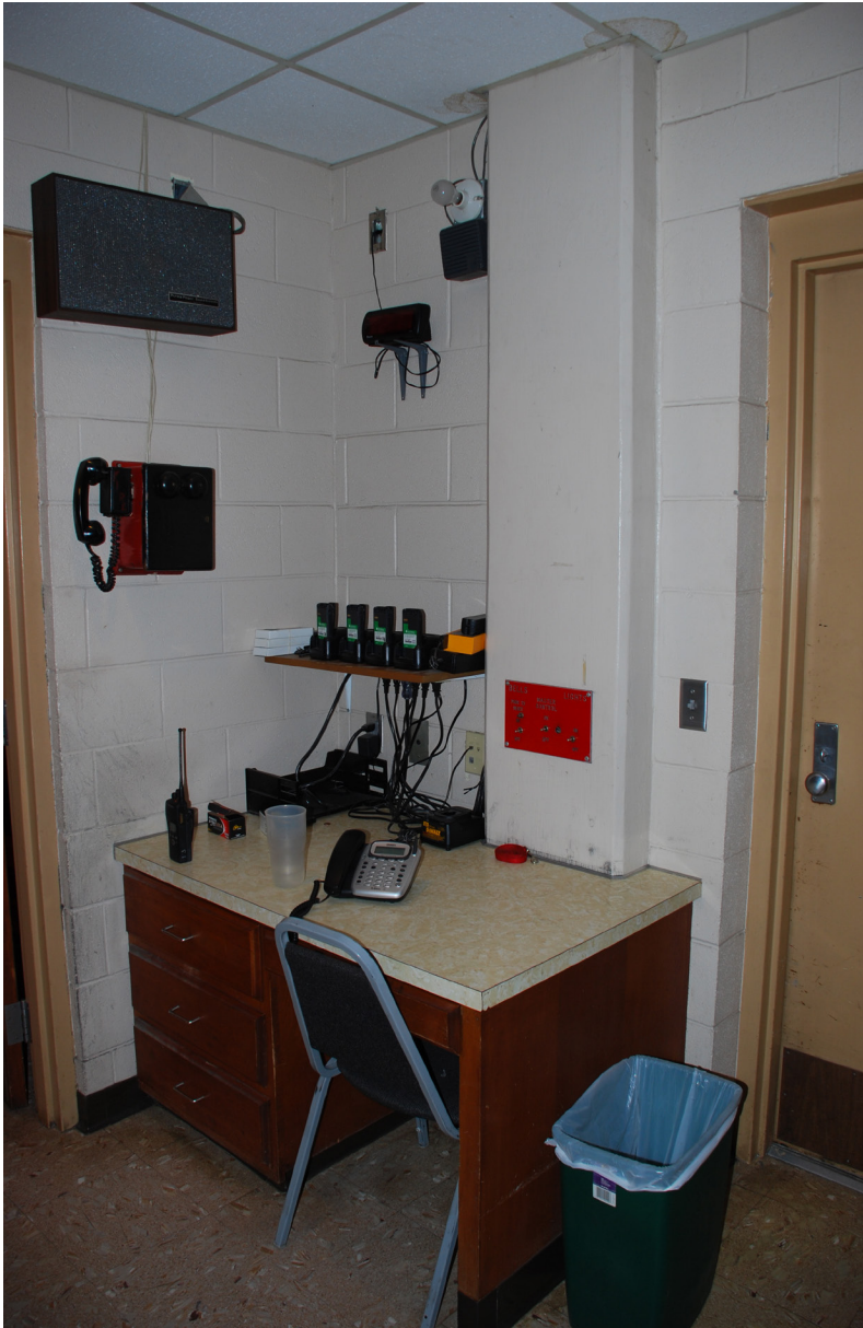
The desk in the SW corner of the dorm is used for communication equipment and radio chargers. The exit door should have a push bar rather than a door knob style latch to make a quick exit smoother for firefighters responding to calls. Note that the trash can is in the path of travel.
