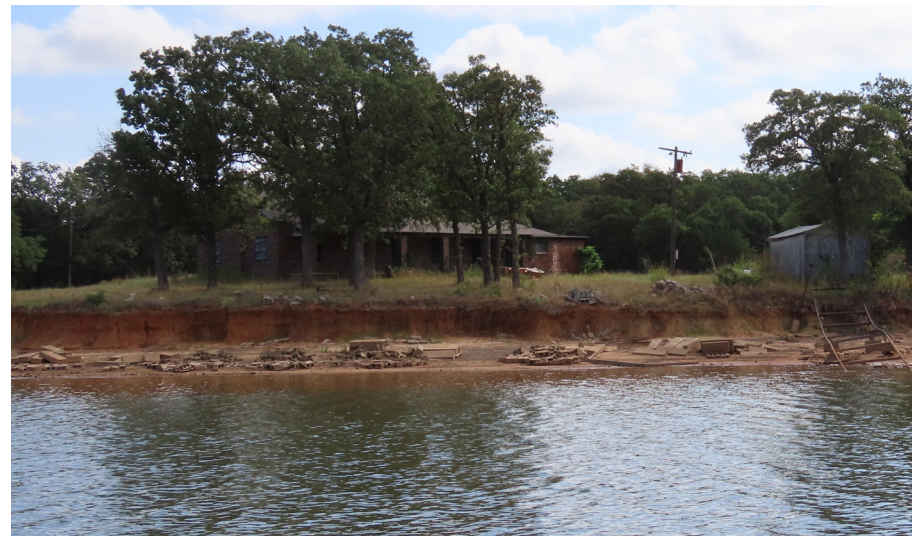
Failed seawalls create hard edges that are susceptible to waves and currents. This can endanger properties and structures and increase erosion rates.
