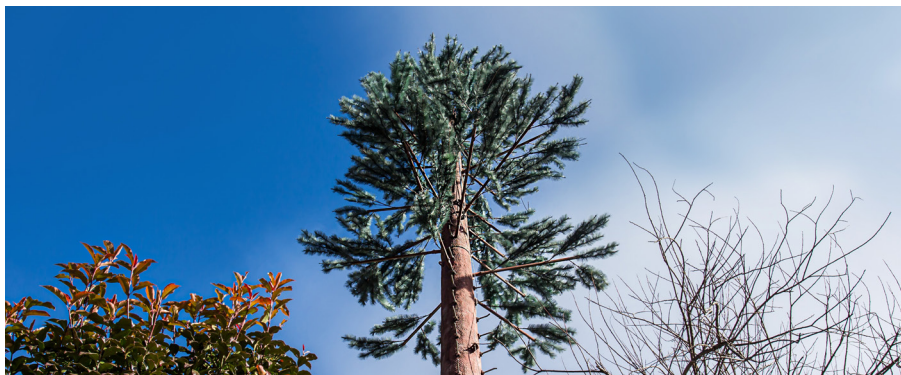
Telecommunication towers can be designed as trees to be camouflaged into the natural environment.
