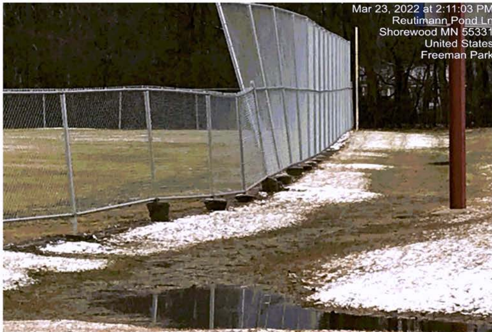
Figure 1 – Freeman Fence Heaving
