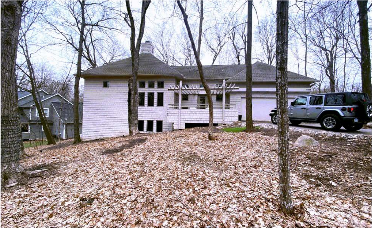
4805 Rustic Way - North Façade
