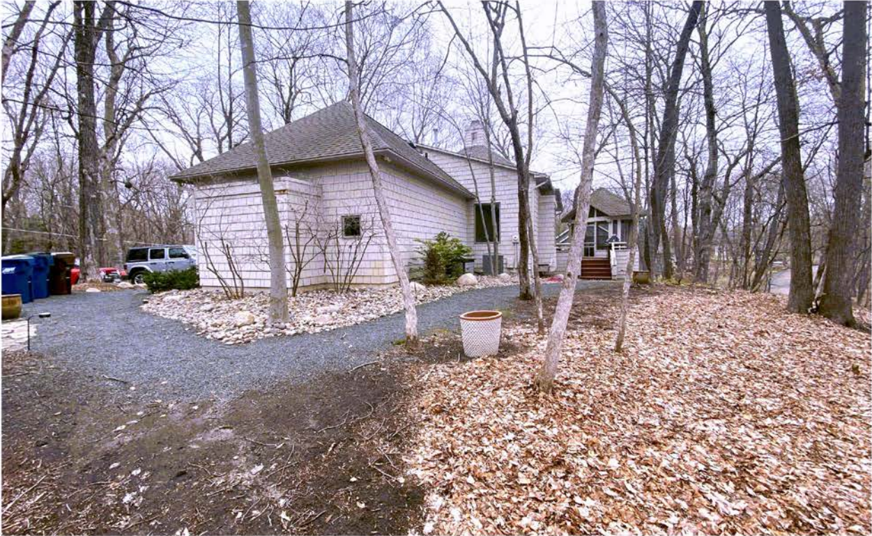
4805 Rustic Way - West Façade
