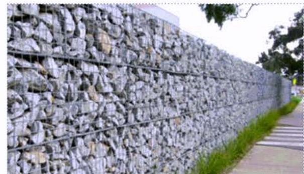
Examples of gabion walls provided by the applicant
