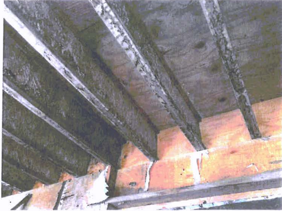
A-61: VIEW OF FLOOR JOISTS SAME AREA
