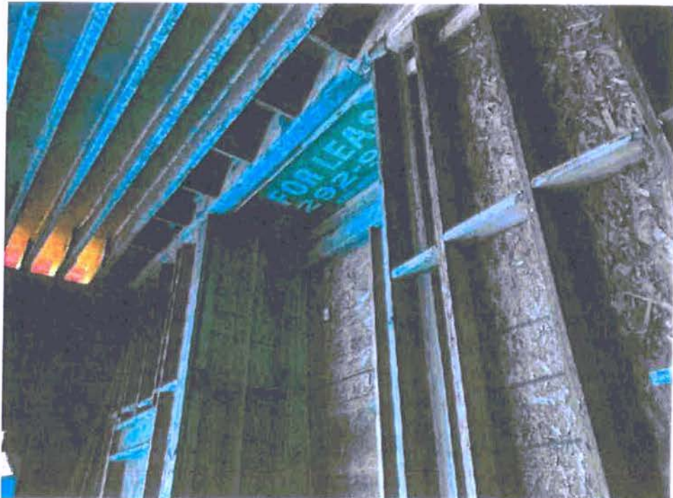
A-92: SOUTH WALL IN GARAGE
