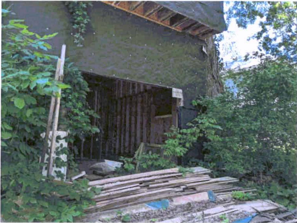
Photograph 11: West side exterior of garage addition.
