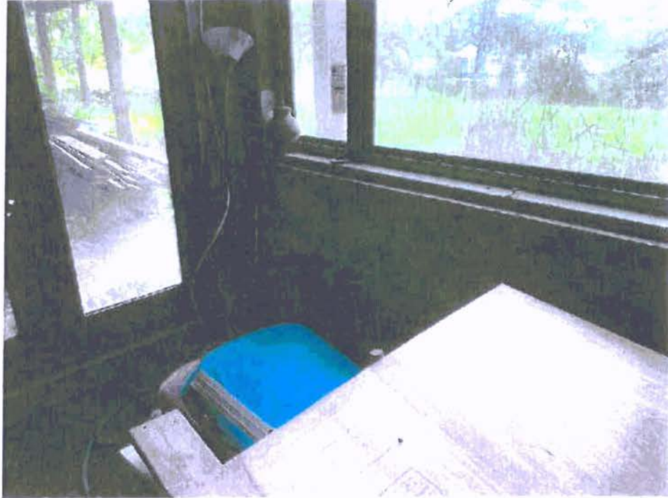
A-83: SOUTHEAST CORNER NEAR DOOR
