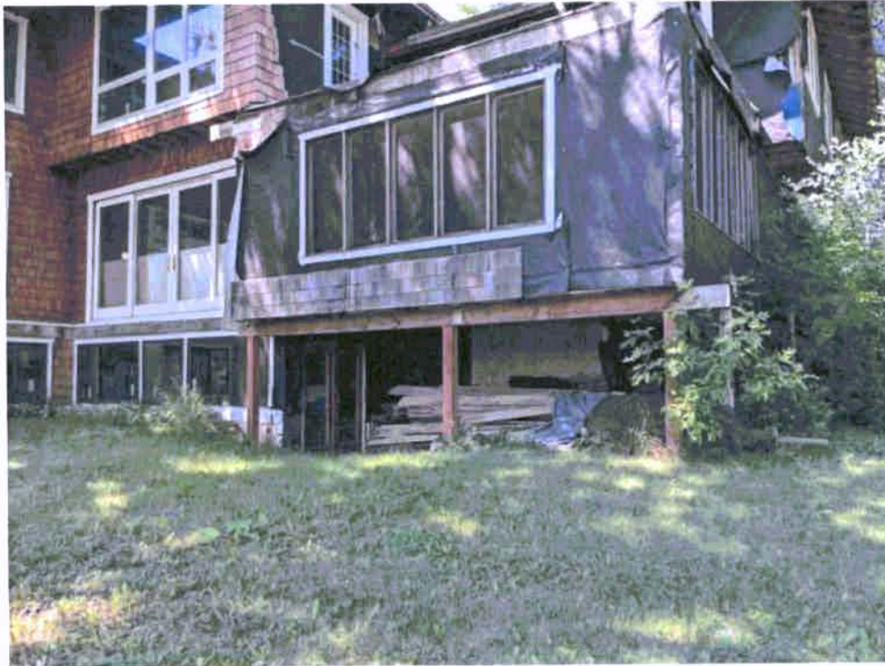
Photograph 6: South exterior of porch addition.
