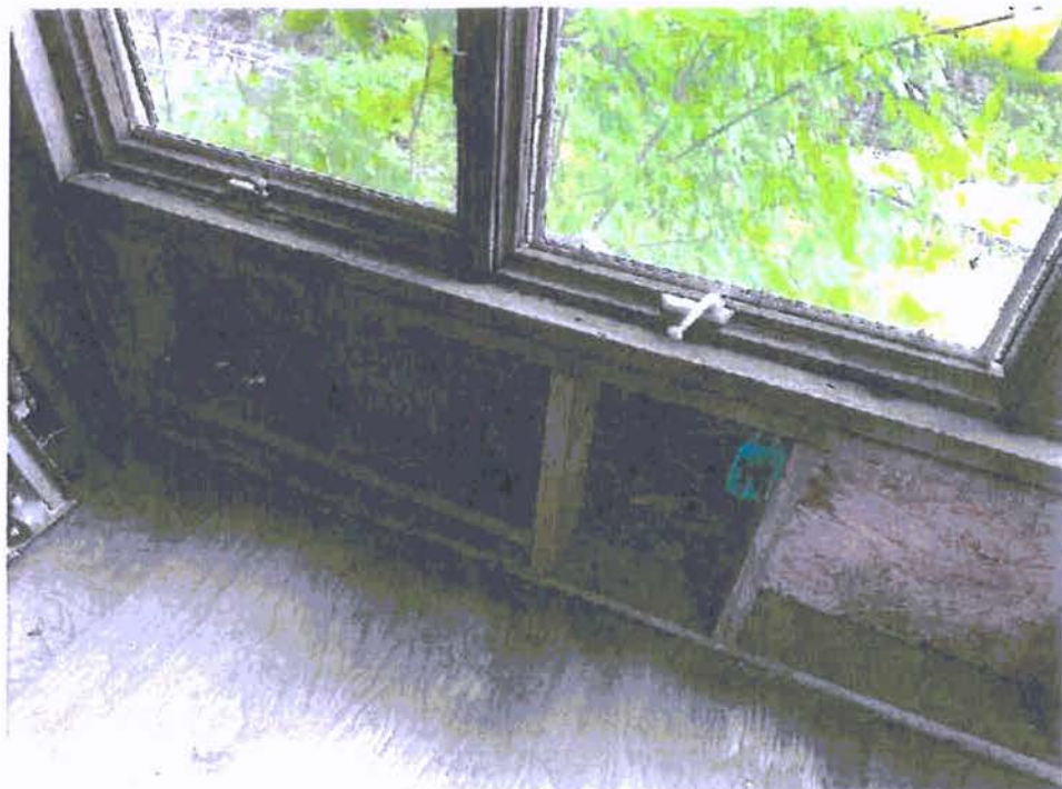
A-70: VIEW OF SHEATHING BELOW EAST WINDOWS
