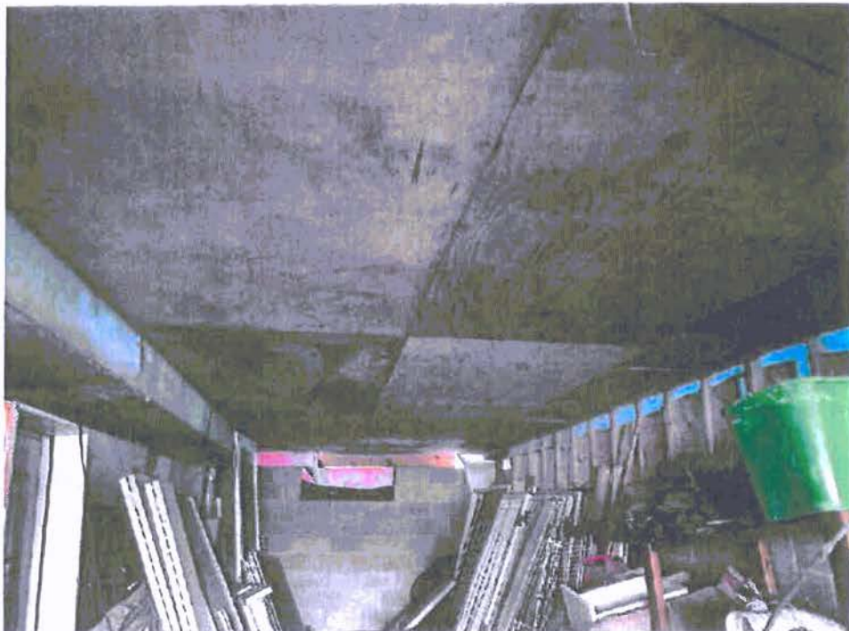
A-86: UNDERSIDE OF ORIGINAL PORTION OF HOME
