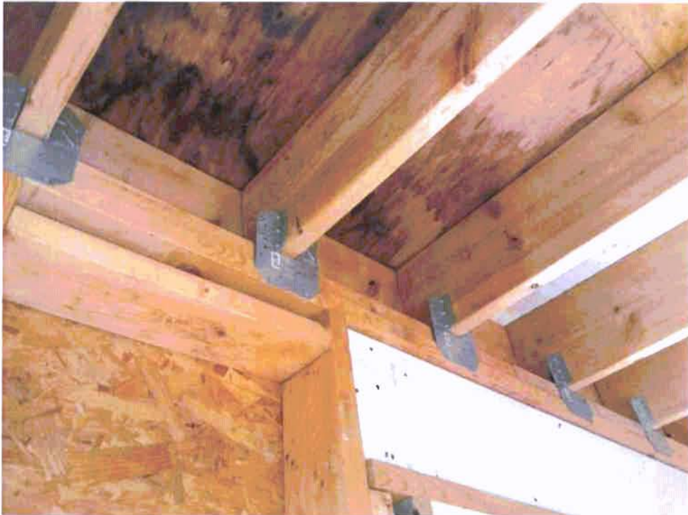
Photograph 10: Unattached beams supporting second floor (2019).
