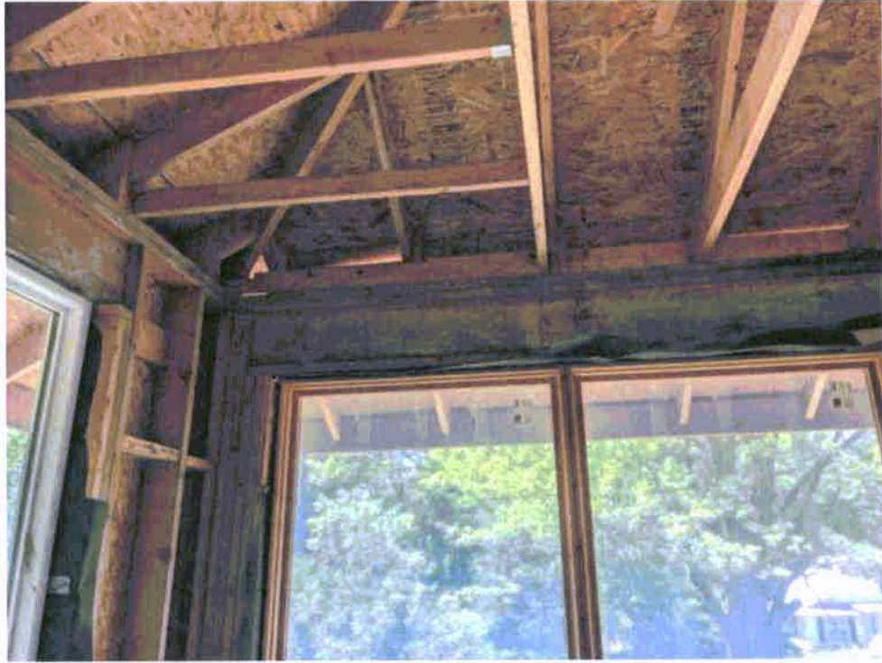
Photograph 24: Interior roof framing in second floor addition.
