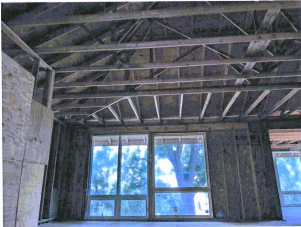
Photograph 29: Interior of second floor addition.
