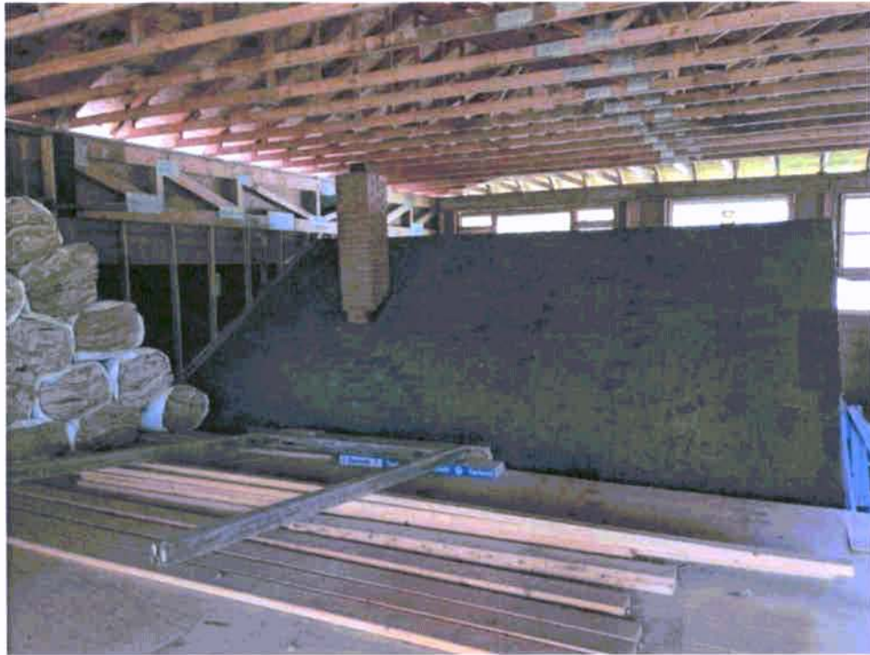
Photograph 21: Interior of second floor addition with original structure visible.
