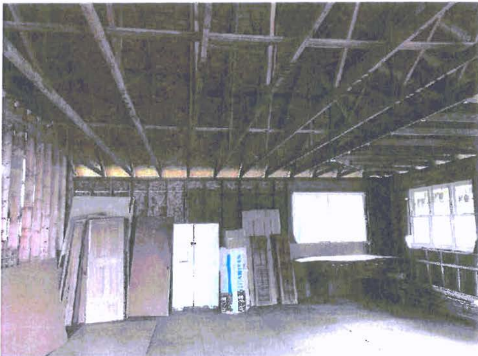
A-26: NORTH WALL, EAST QUADRANT OVER GARAGE
