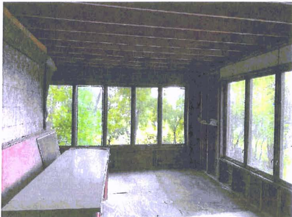
A-68: EAST WALL IN PORCH
