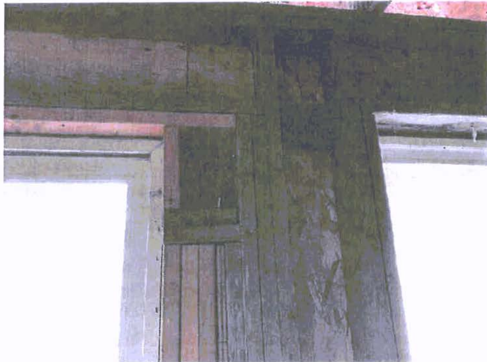
A-46: FRAMING ALONGSIDE WINDOW IN SOUTH WALL
