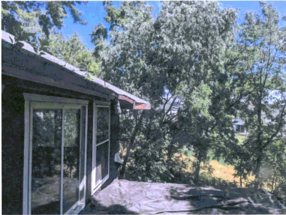
Photograph 21: Exterior of second floor addition.
