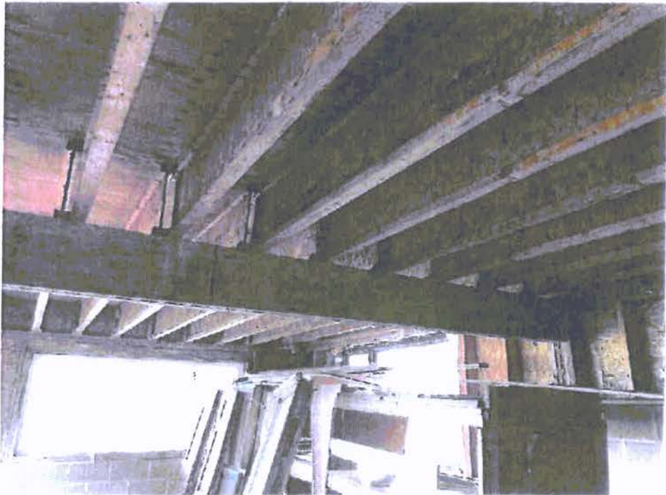
A-80: VIEW OF HEADER SUPPORTING MAIN FLOOR JOISTS AT SOUTHWEST QUADRANT
