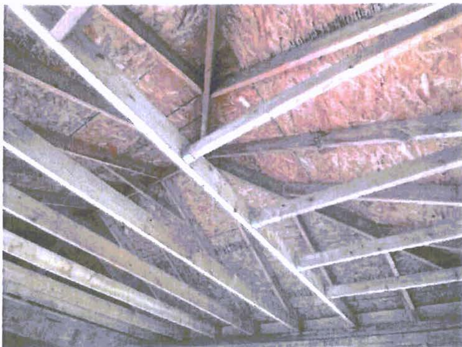
A-20: VIEW OF HIP ROOF FRAMING AT SOUTHWEST QUADRANT OF HOME
