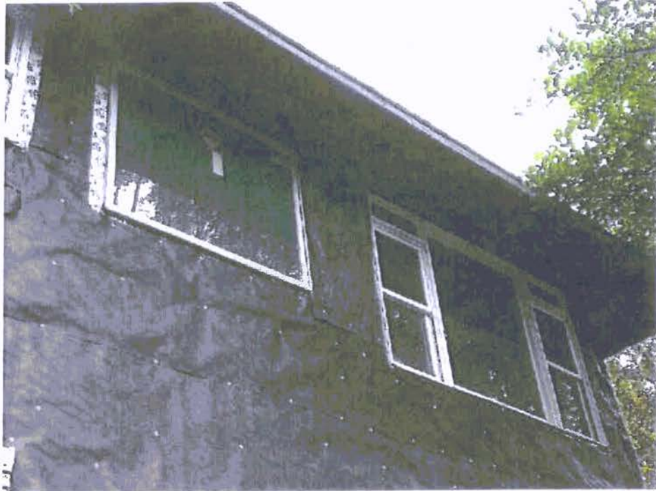
A-15: ADJACENT WINDOWS AT NORTH SIDE, UPPER LEVEL
