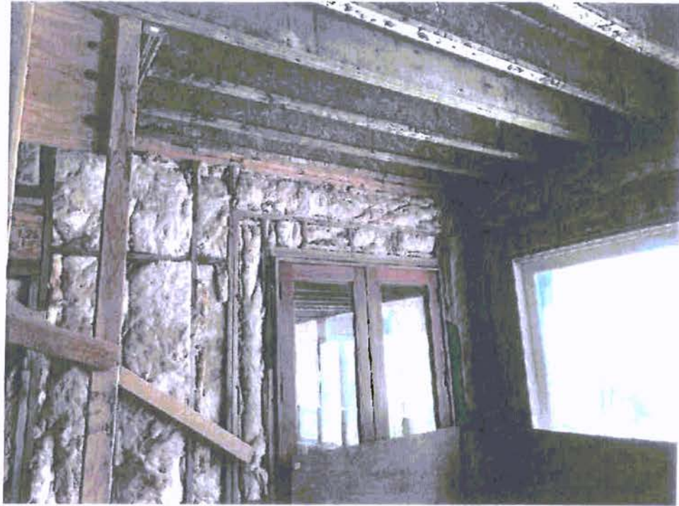
A-63: EAST WALL, DOOR TO PORCH
