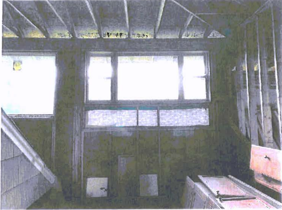
A-23: NORTH WALL, CENTRAL QUADRANT
