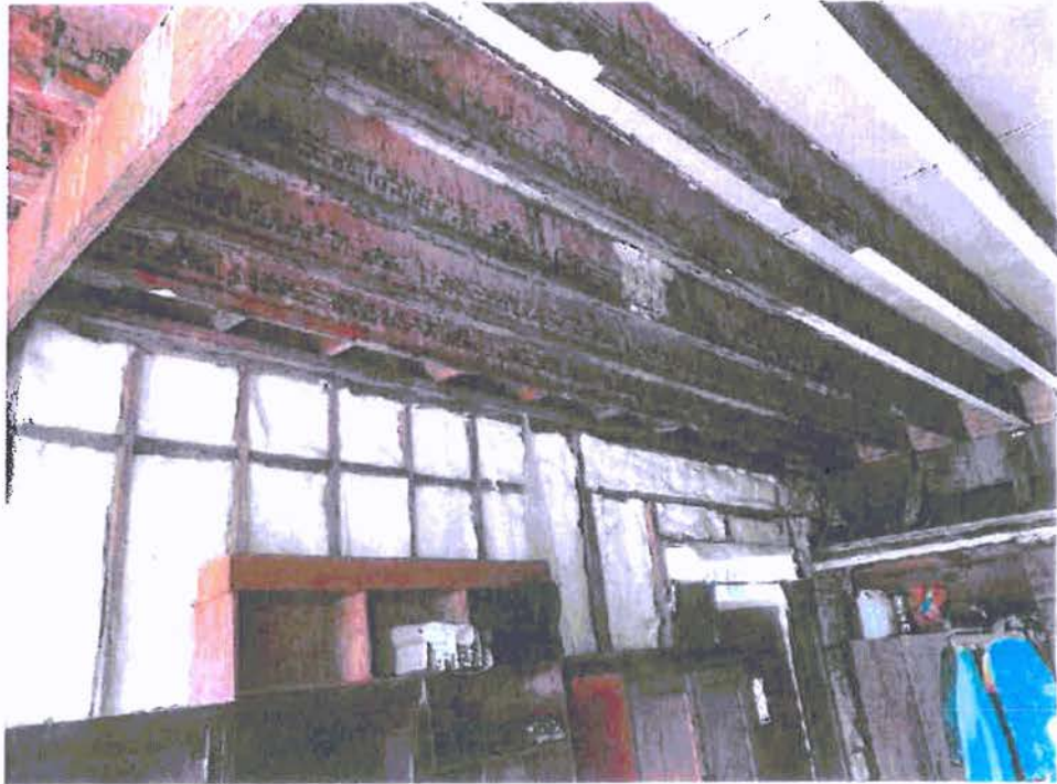
A-56: WEST WALL SOUTH OF ENTRY DOOR
