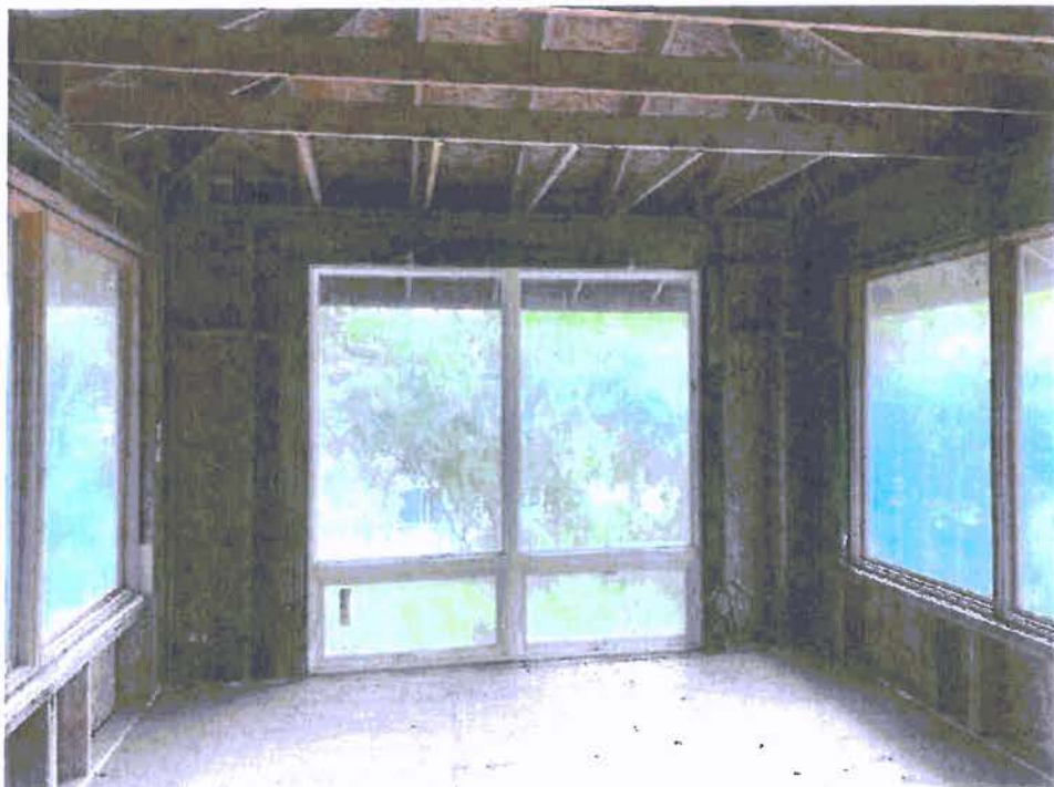
A-18: SOUTH WALL, SOUTH UPPER LEVEL AT SOUTHWEST QUADRANT
