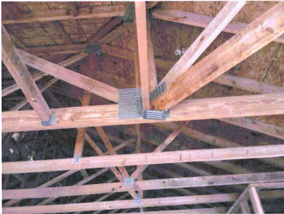
Photograph 7: Roof truss connection (2022).
