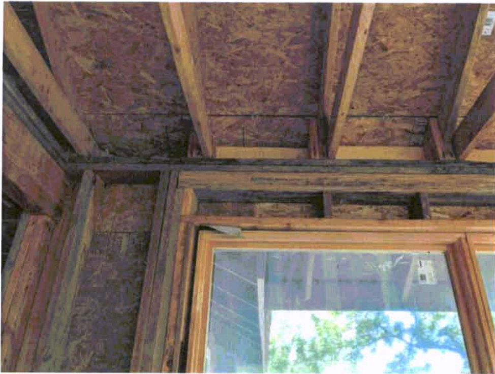
Photograph 26: Interior window framing of second floor addition.
