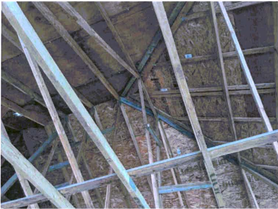
Photograph 19: Roof framing of second floor addition.
