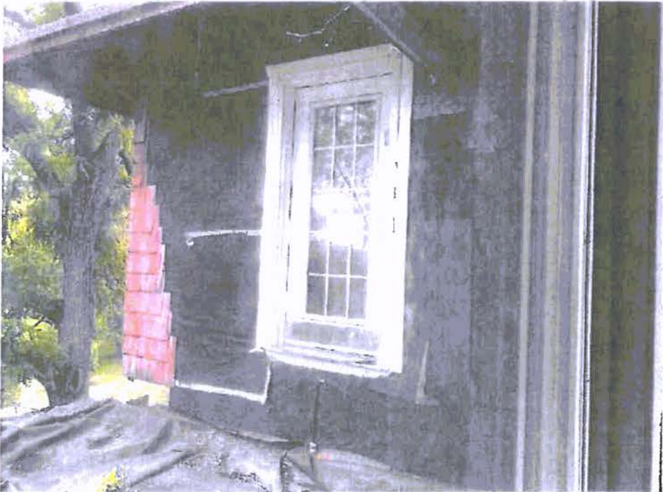
A-34: DOOR IN EAST WALL AT UPPER PORCH ROOF ACCESS
