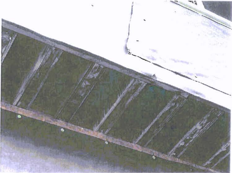
A-11: VIEW OF CANTILEVER FLOOR JOISTS AT UPPER LEVEL, EAST SIDE
