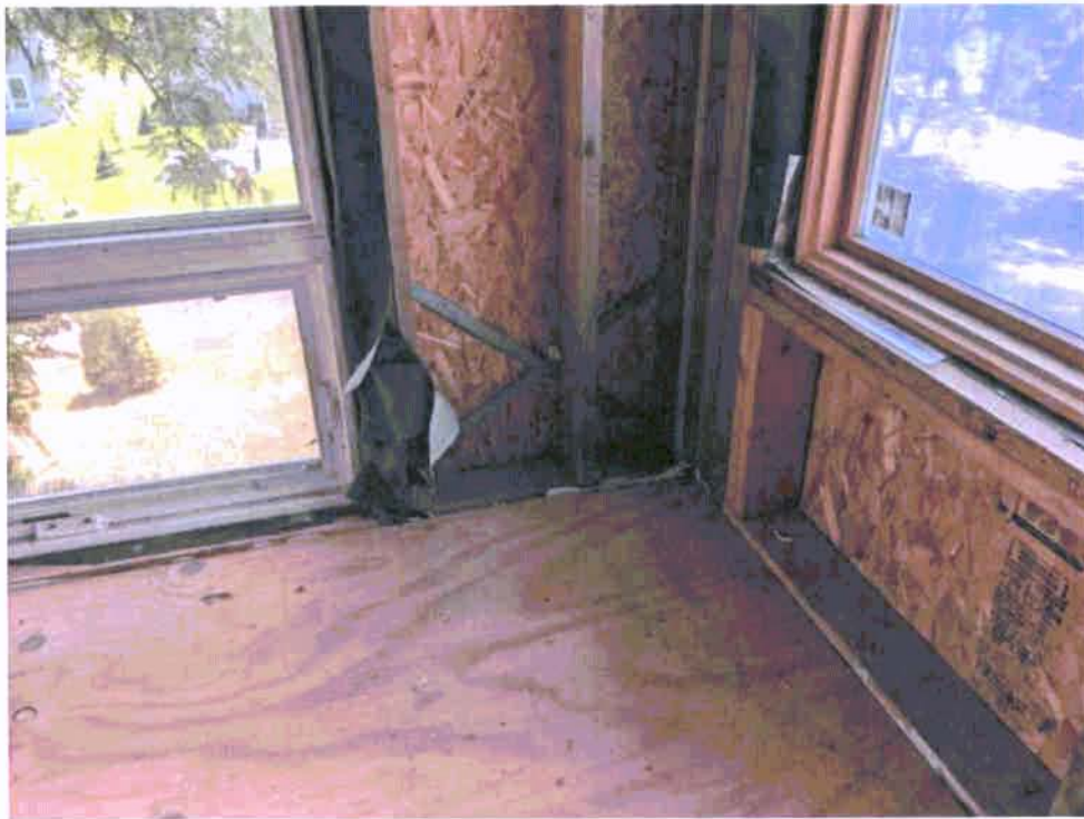
Photograph 25: Interior wall framing of second floor addition.
