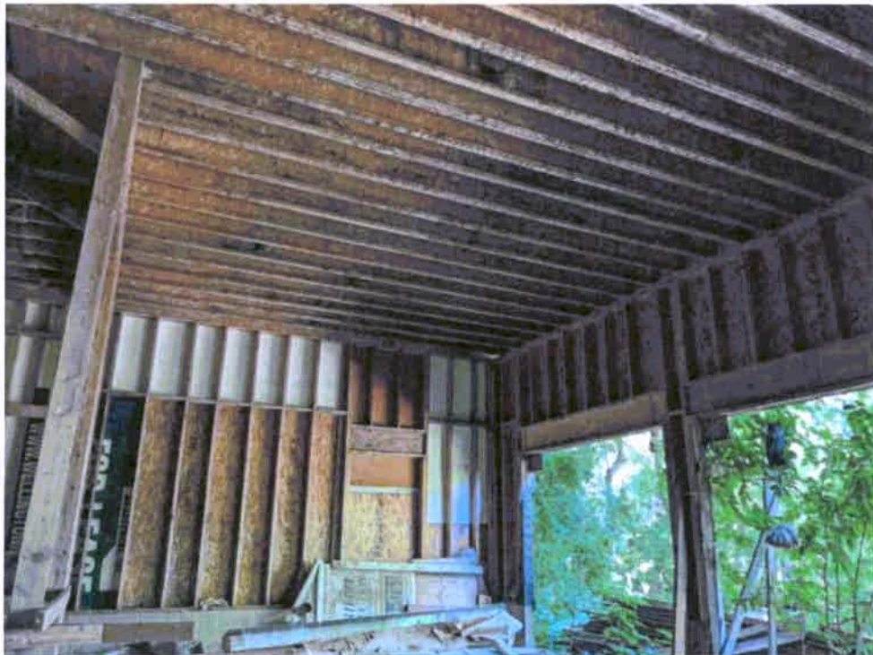
Photograph 8: Interior of garage addition.
