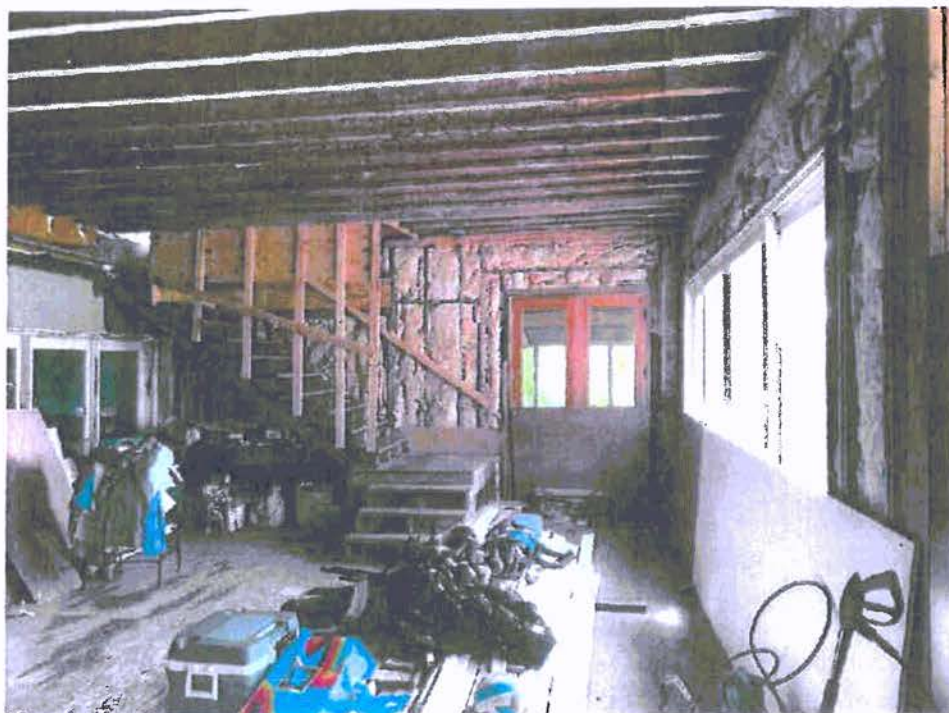
A-58: VIEW EAST TOWARDS STAIRWAY
