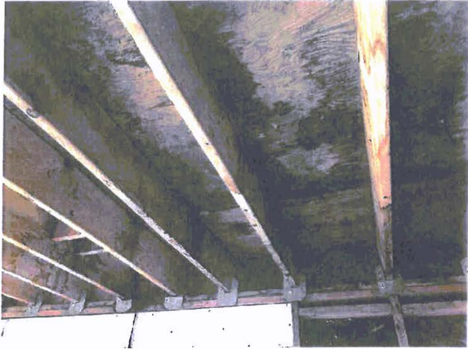
A-69: VIEW OF ROOF FRAMING AT PORCH STRUCTURE
