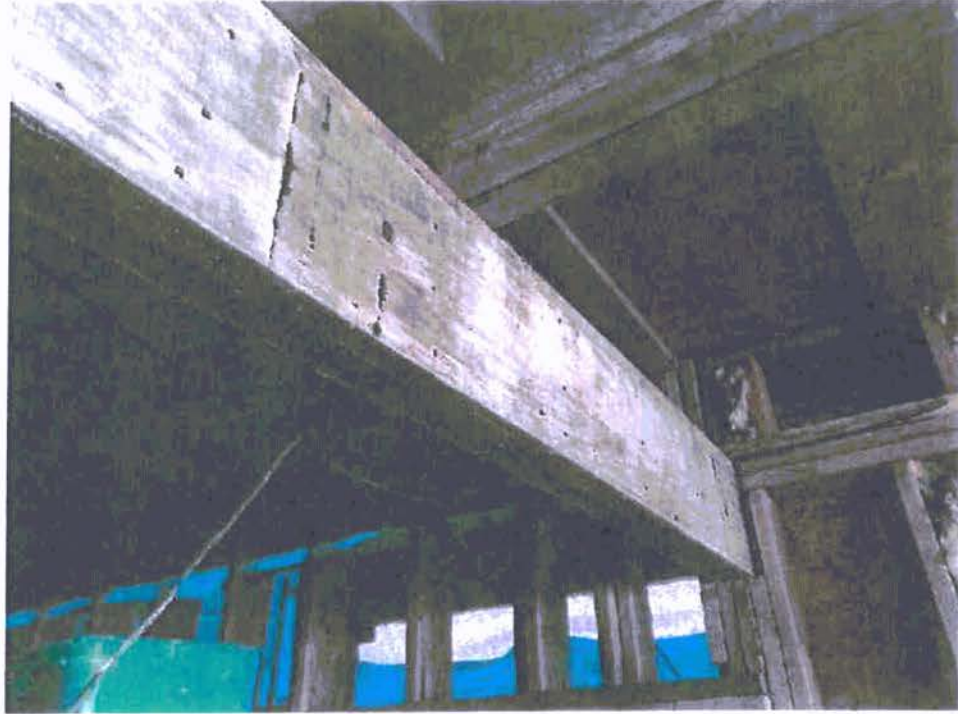
A-85: VIEW OF HEADER AT LOWER LEVEL UNDER AREA OF STAIRWAY
