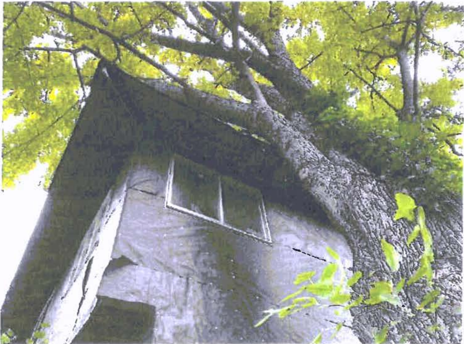
A-12: NORTHEAST CORNER AT UPPER LEVEL
