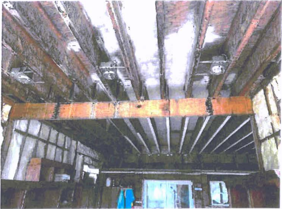
A-55: VIEW OF EXISTING HEADER SUPPORTING UPPER FLOOR JOISTS
