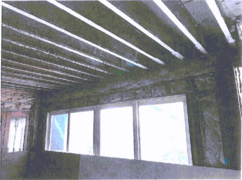
A-59: SOUTH WALL, 16 FOOT OPENING FOR DOOR UNIT
