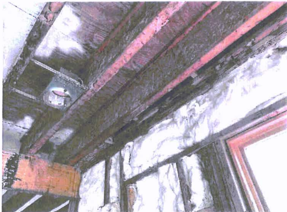
A-54: VIEW OF FRAMING AT EAST WALL
