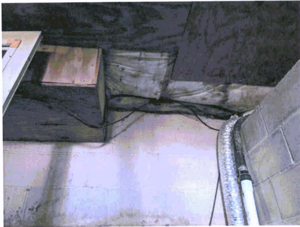
Photograph 14: Basement ceiling of structure at existing structural foundation wall.
