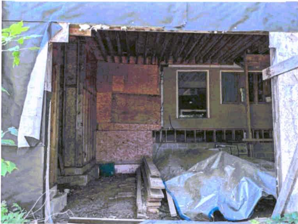
Photograph 12: Interior of garage addition.
