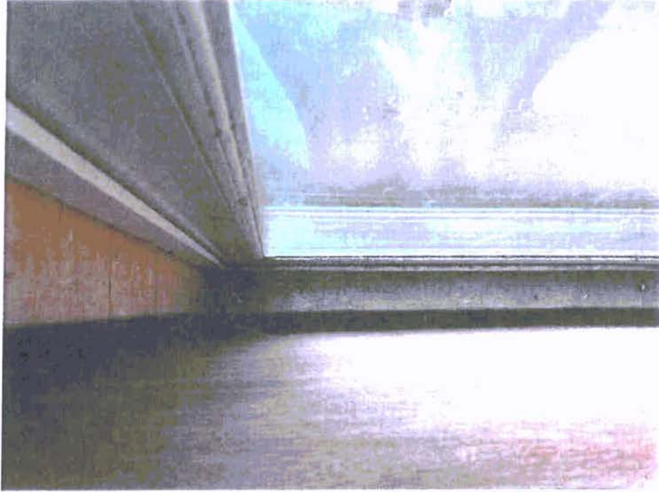
A-41: SILL OF EAST WINDOW IN SOUTH WALL, SOUTHEAST QUADRANT
