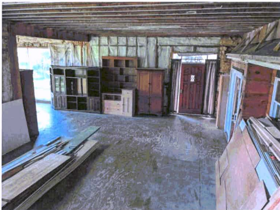
Photograph 31: Interior of first floor addition.
