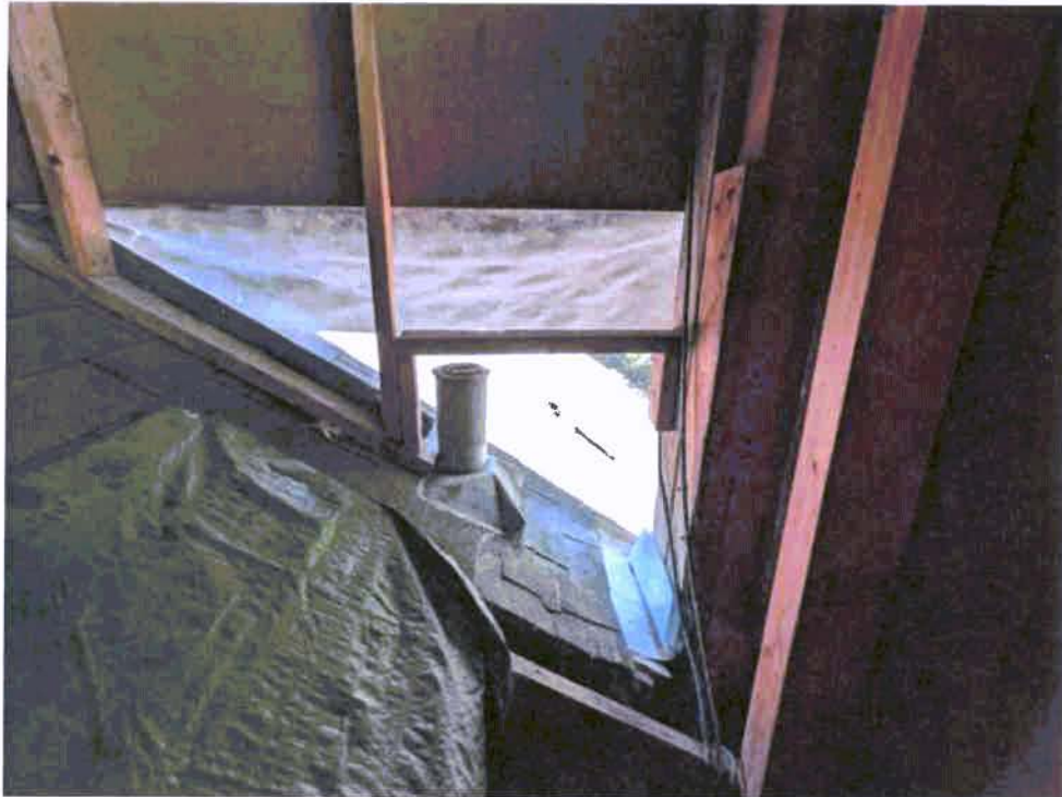
Photograph 27: Exterior wall framing above existing structure.
