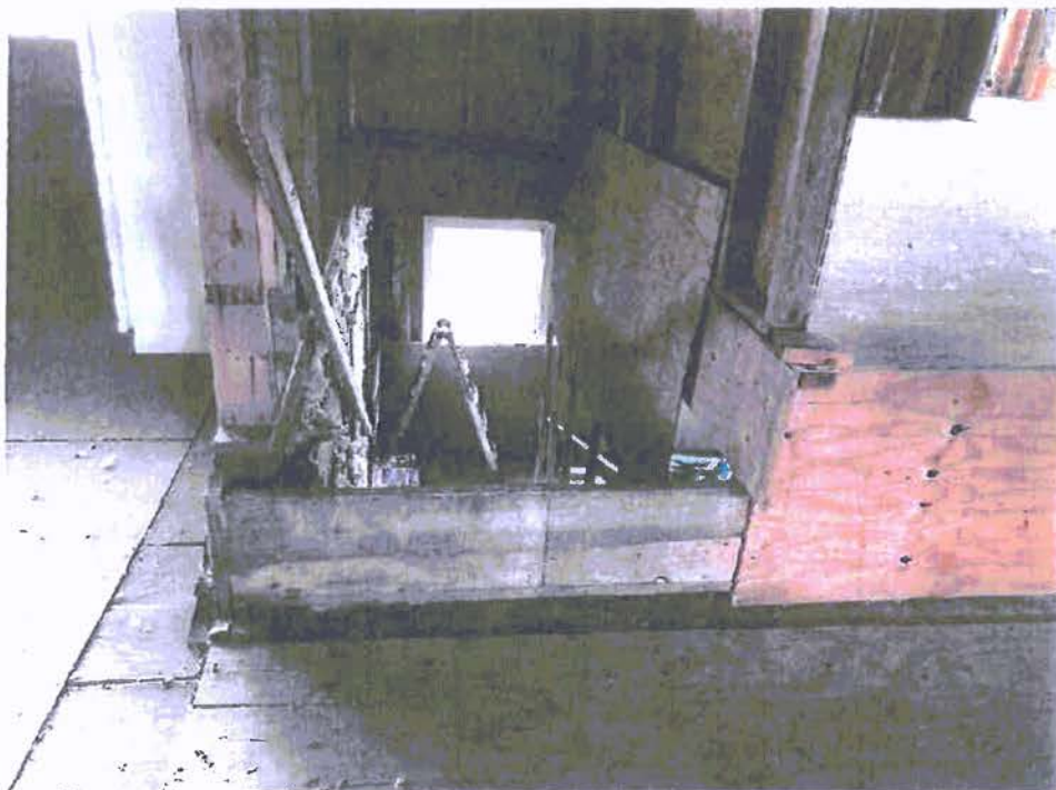
A-66: TOP OF STAIRWAY, HEADER EXTENDS TO LEFT BEARING WALL
