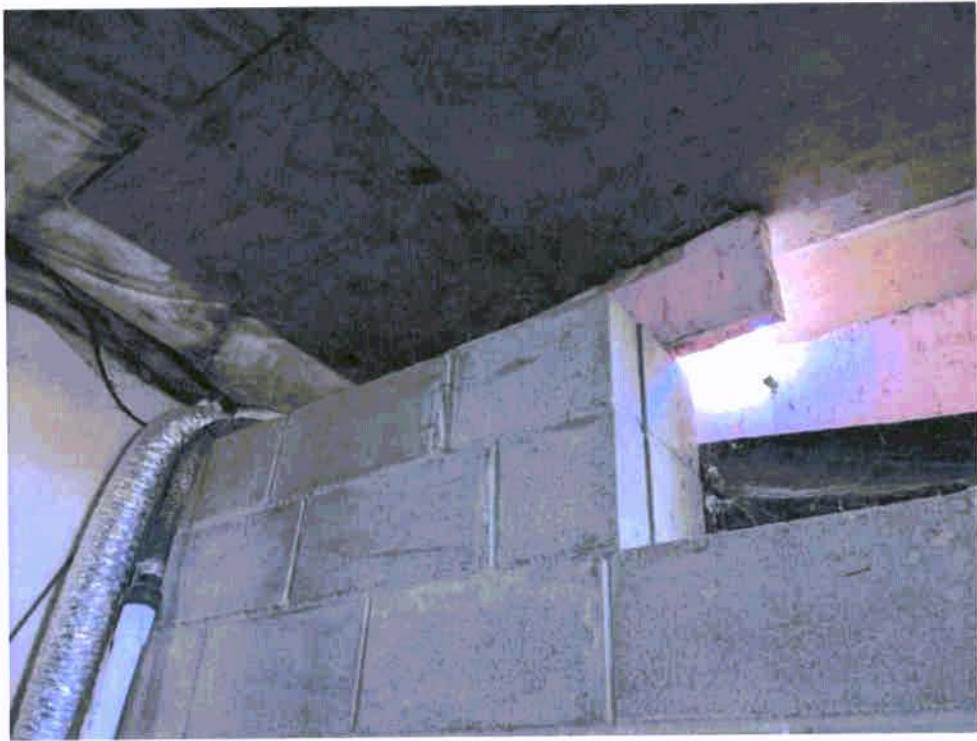
Photograph 13: Basement wall of structure.
