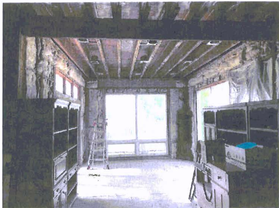
A-48: MAIN LEVEL, VIEW SOUTH AT WEST PORTION
