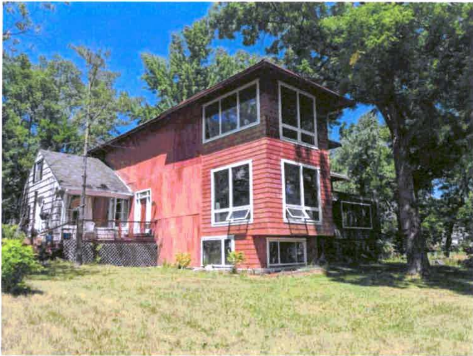
Photograph 3: Southwest corner exterior of the house.
