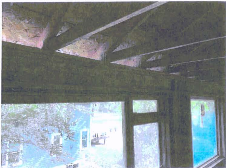
A-38: VIEW ALONG TOP OF WINDOW
