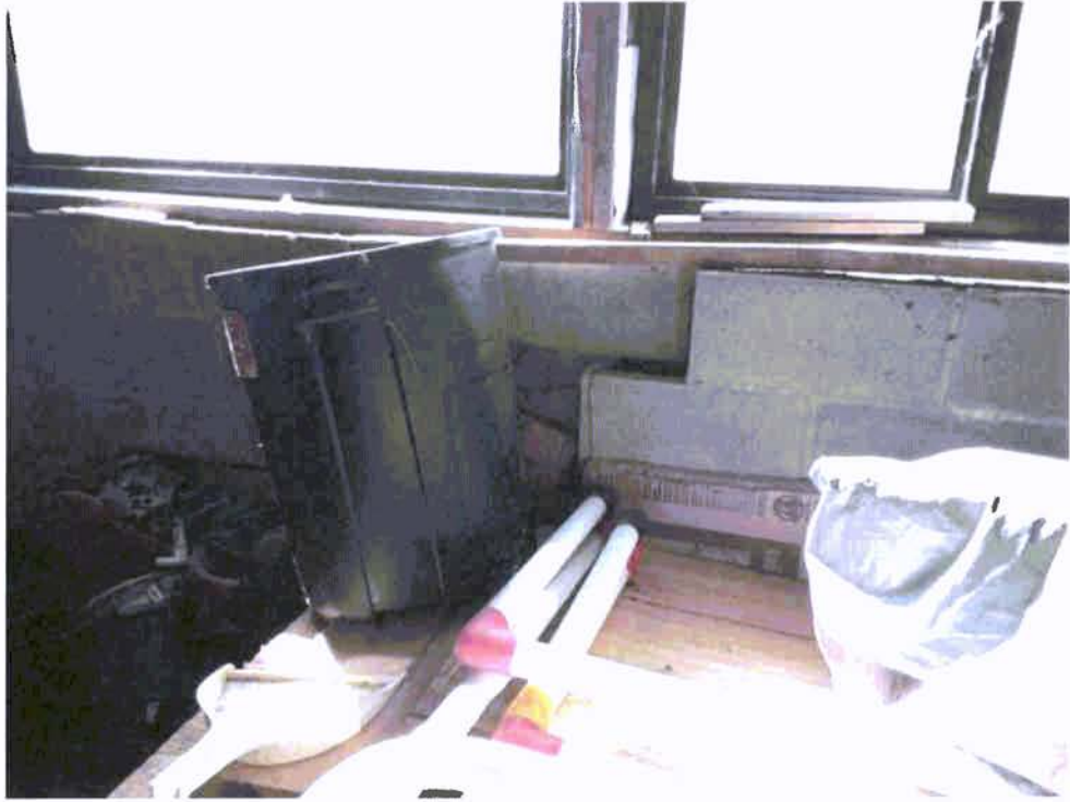
Photograph 13: Variation of foundation wall thickness (2019).
