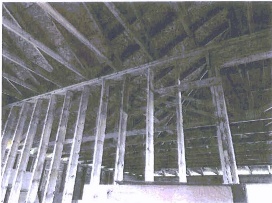
A-24: CENTER BEARING WALL SUPPORTING TRUSSES
