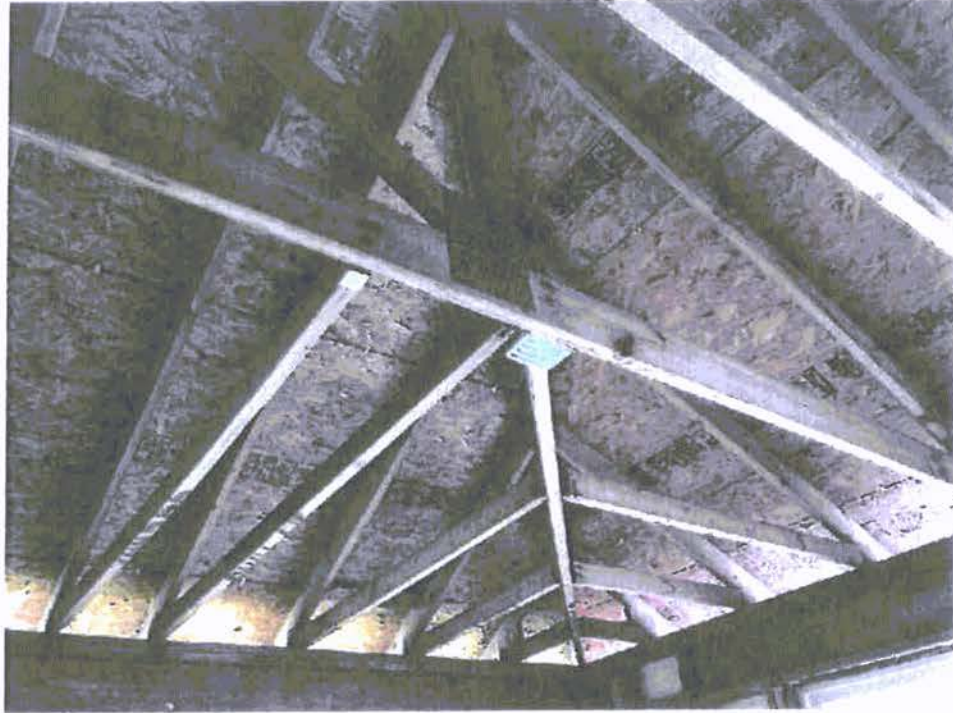
A-29: VIEW OF FRAMING AT HIP ROOF TRANSITION
