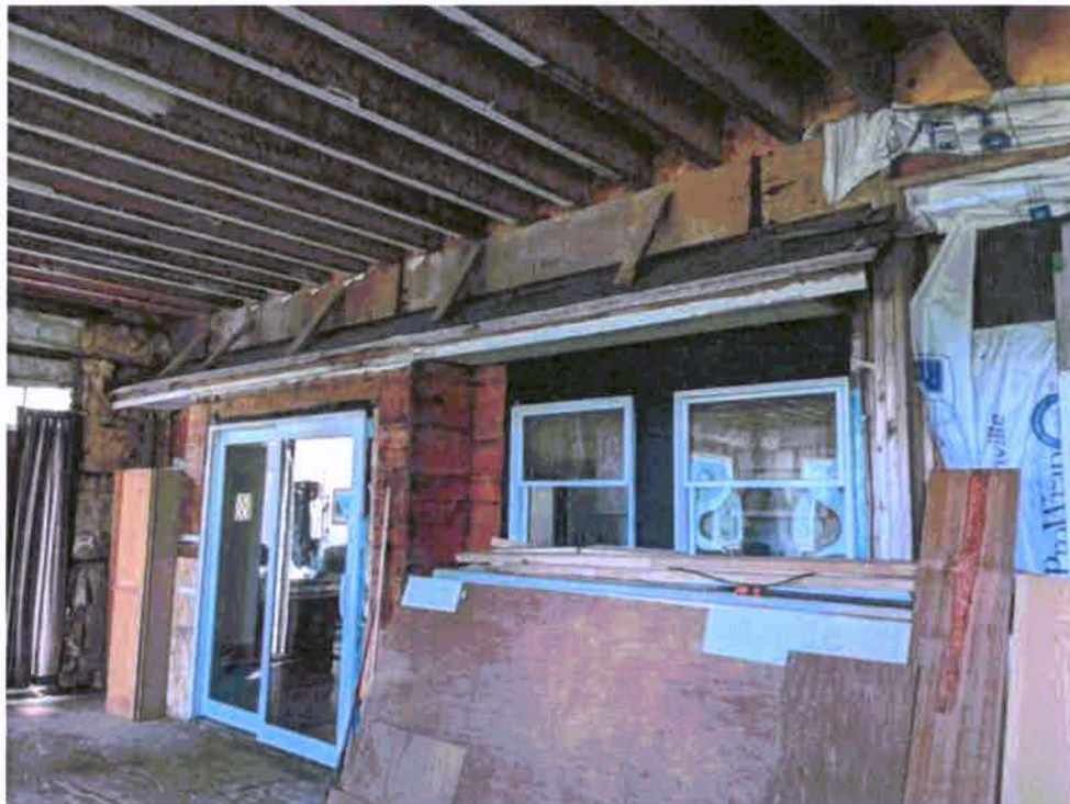
Photograph 16: Interior of front porch addition.
