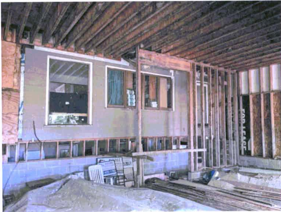
Photograph 10: Interior of garage addition.
