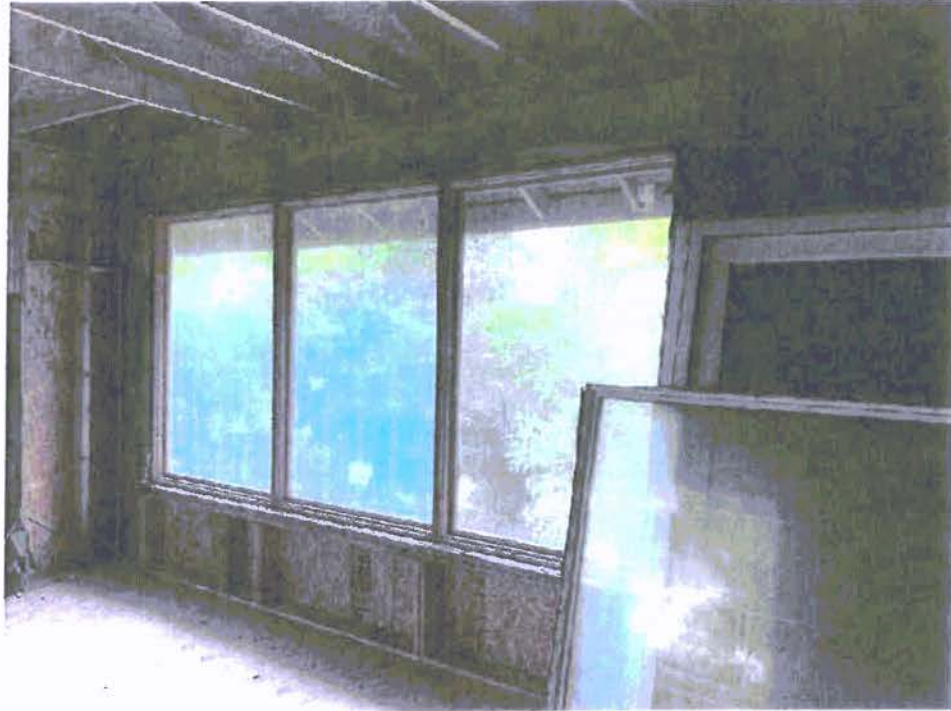
A-17: UPPER LEVEL, WEST WINDOW AT SOUTHWEST QUADRANT
