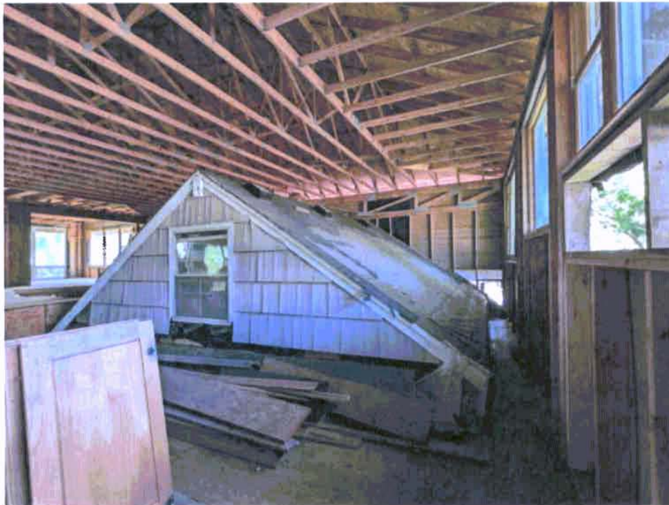
Photograph 8: Added loading and modifications to original structure (2022).
