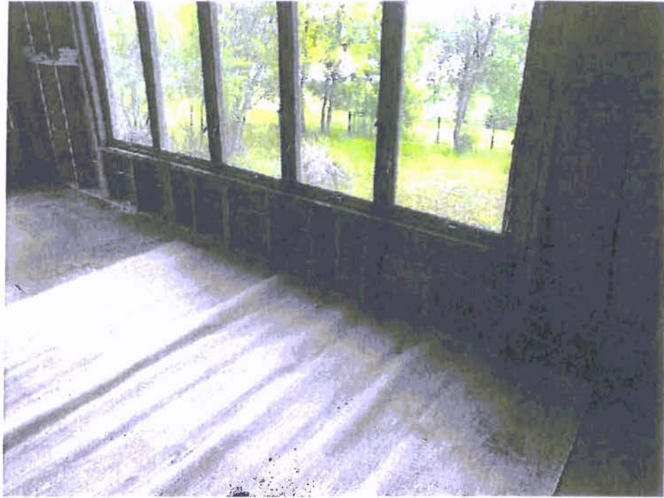
A-67: SOUTH WALL IN PORCH
