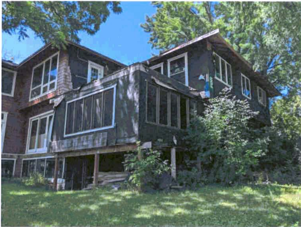
Photograph 7: Southeast corner exterior of structure.
