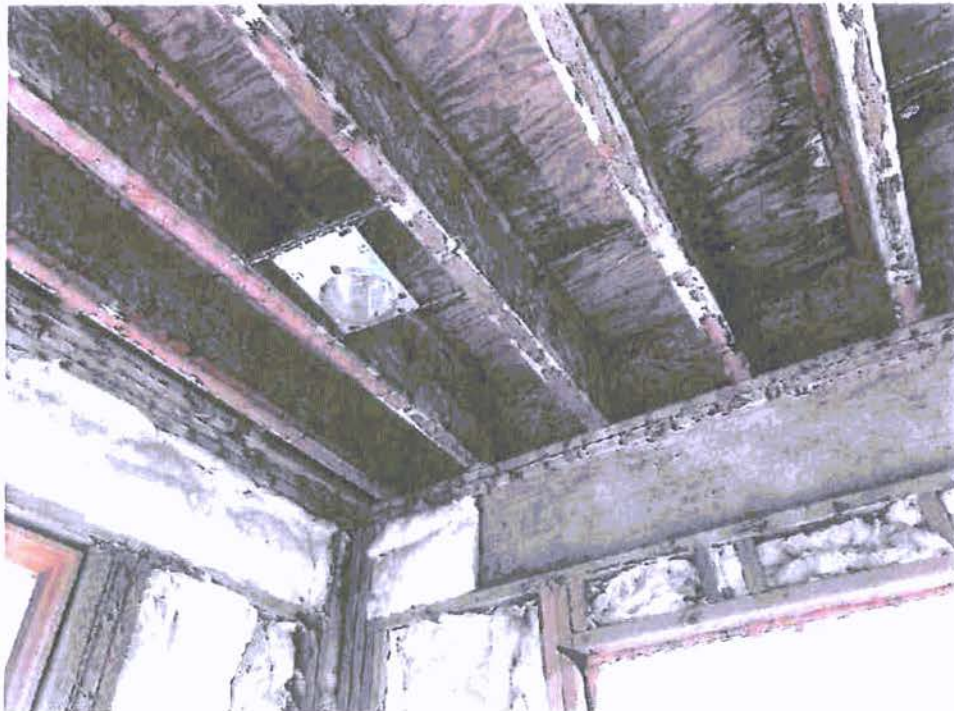
A-52: SOUTHEAST CORNER AT SOUTHWEST AREA OF HOME
