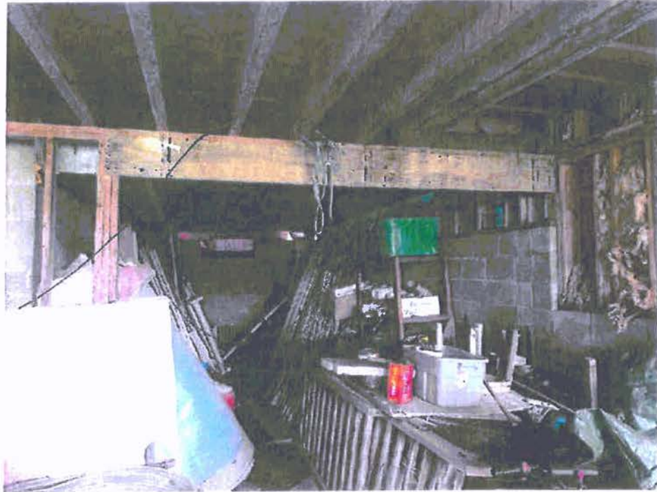
A-75: LOWER LEVEL, VIEW NORTH BEHIND GARAGE
