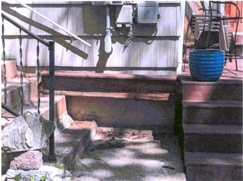
Photograph 14: Front porch addition beam bearing on existing porch step (2022).
