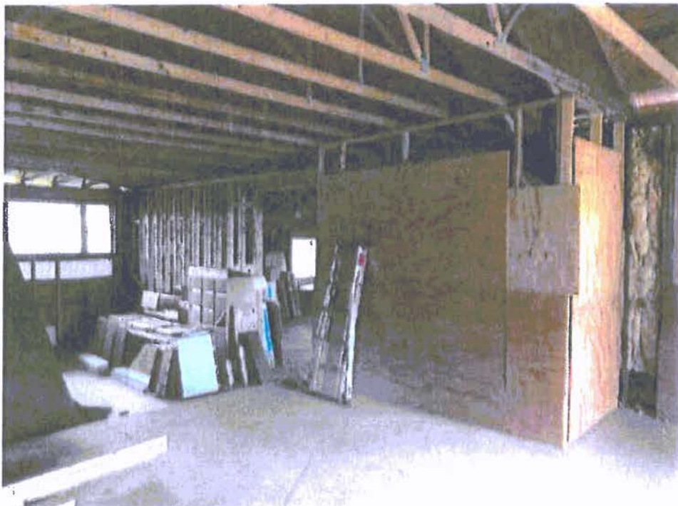
A-22: VIEW EAST AT CENTER BEARING WALL
