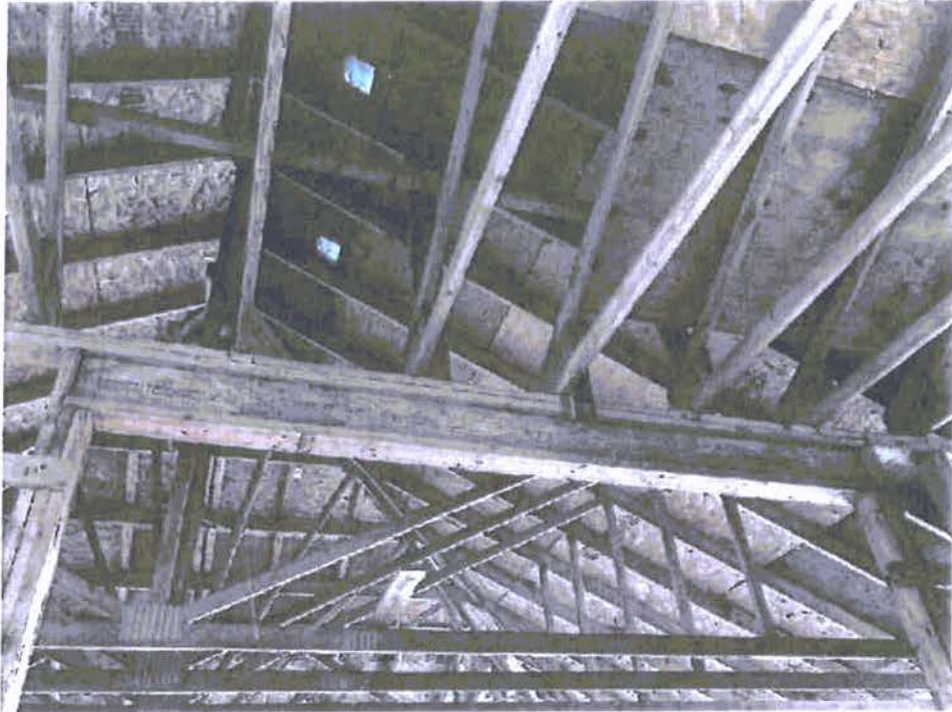
A-25: VIEW OF EXISTING LSL HEADER AT 10 FOOT OPENING
