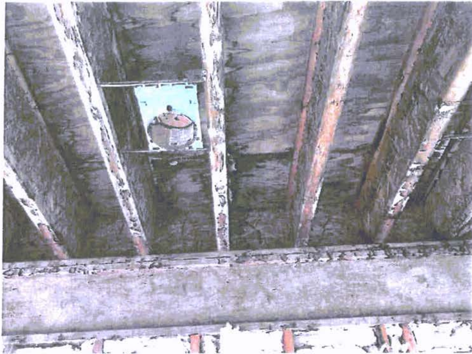
A-51: VIEW OF SUBFLOOR AT SOUTH WALL, CENTRAL QUADRANT
