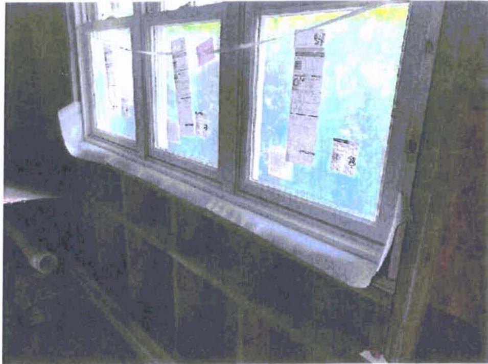
A-45: NORTH WINDOW IN EAST WALL, PAN FLASHING PRESENT
