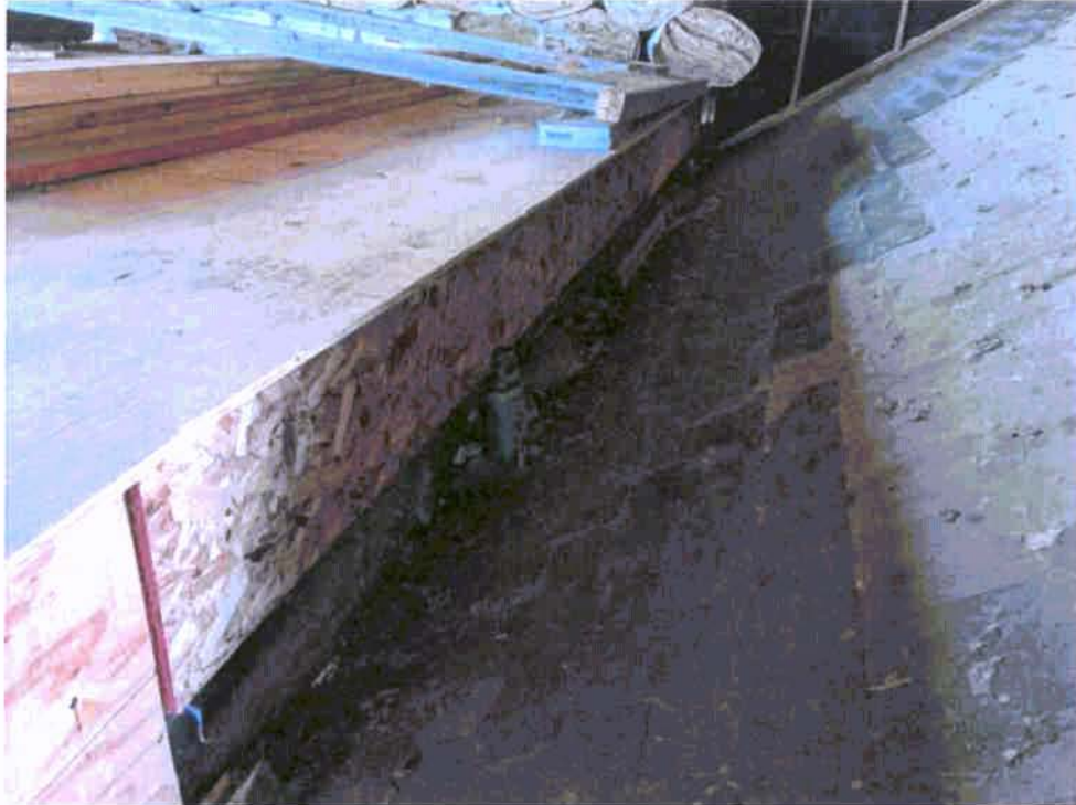
Photograph 30: Framing above existing roof structure.
