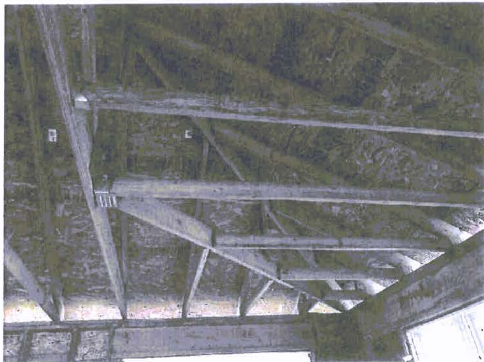
A-30: OPPOSITE END OF WALL SHOWING HIP ROOF FRAMING
