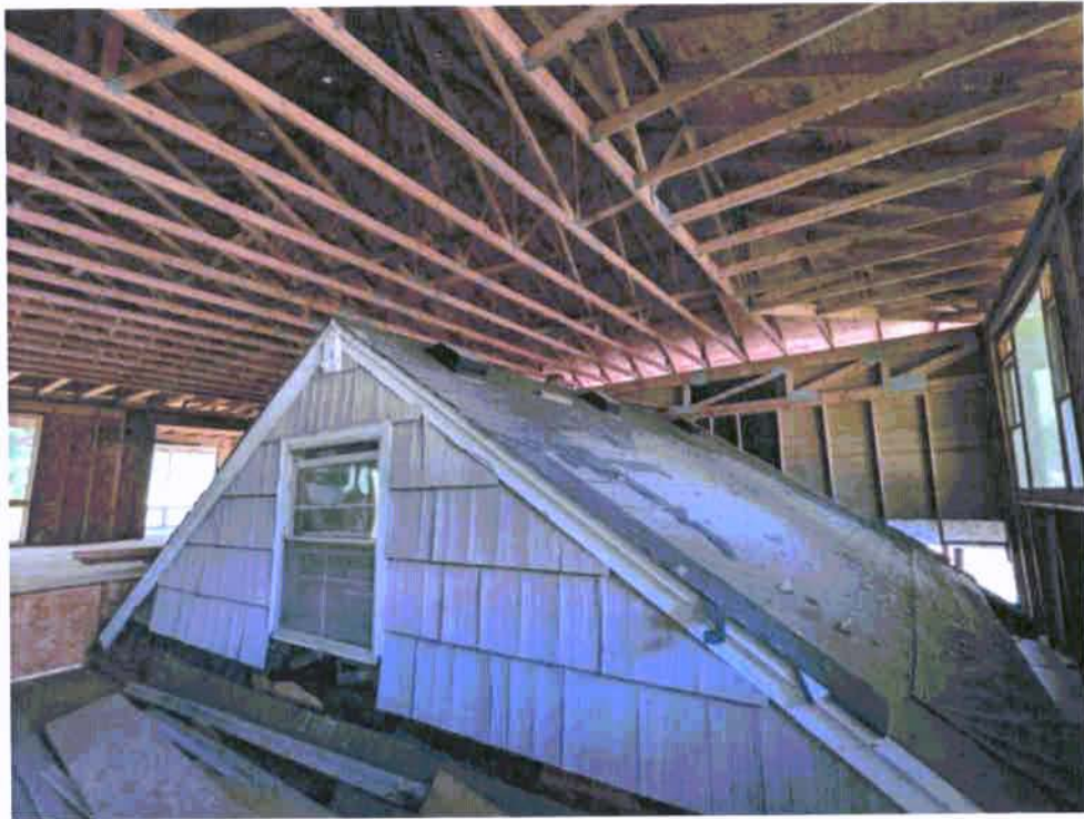
Photograph 28: Interior of second floor addition above original structure.
