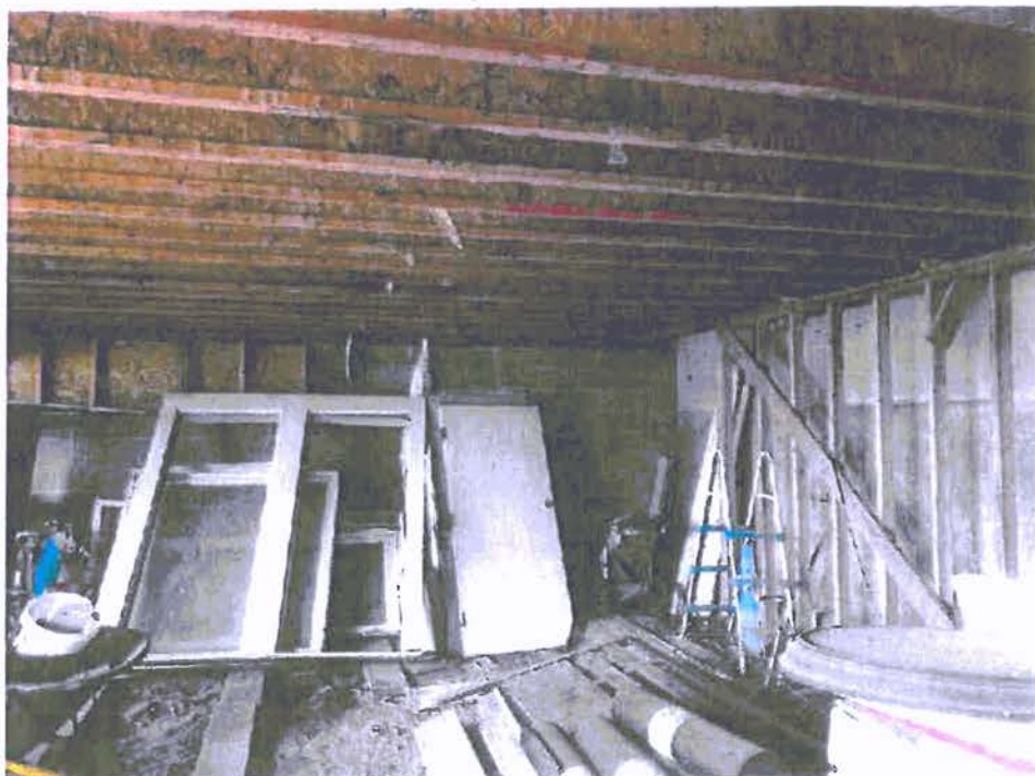
A-76: VIEW WEST AT LOWER LEVEL OF ADDITION
