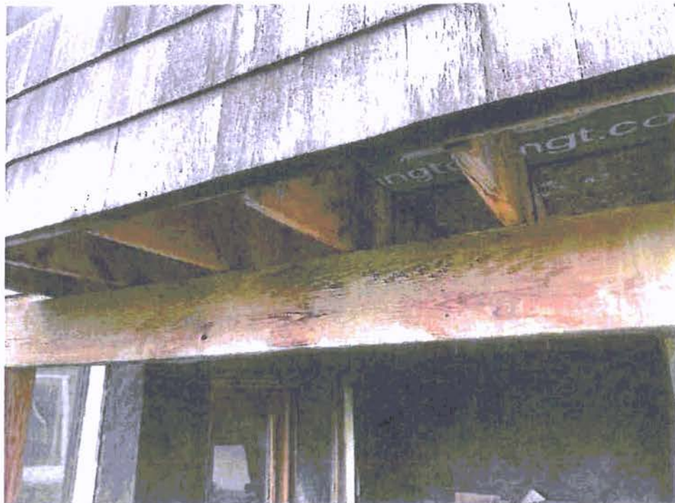
A-8: HEADER AND UNDERSIDE OF FRAMING AT PORCH
