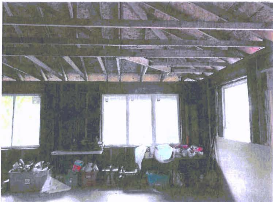
A-28: EAST WALL, SOUTHEAST QUADRANT
