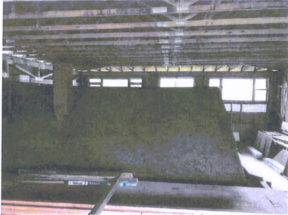
A-21: VIEW NORTH AT WEST QUADRANT OF ADDITION AND ORIGINAL ROOF
