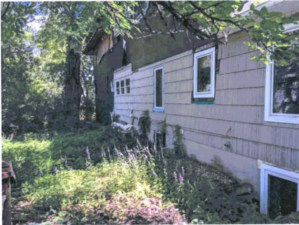
Photograph 2: North side exterior of the house.
