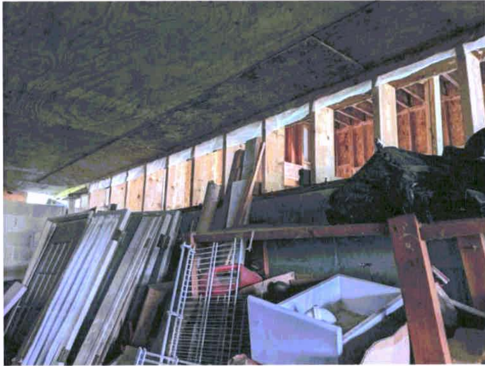
Photograph 3: Cripple lookout wall (2022).
