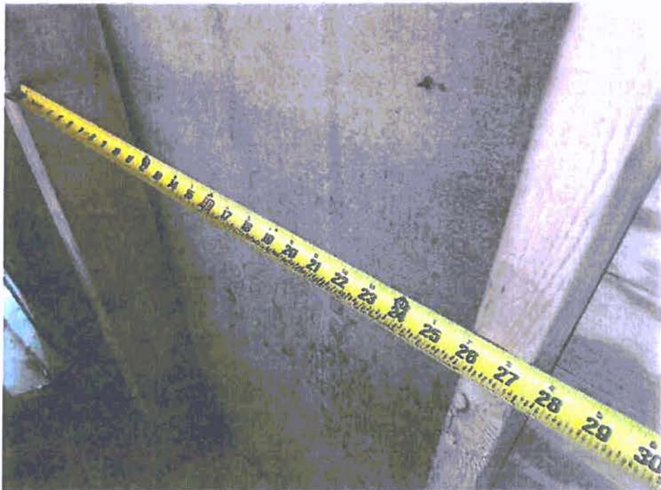
A-40: MEASURE OF EXISTING STUD SPACING UNDER WEST WINDOW
