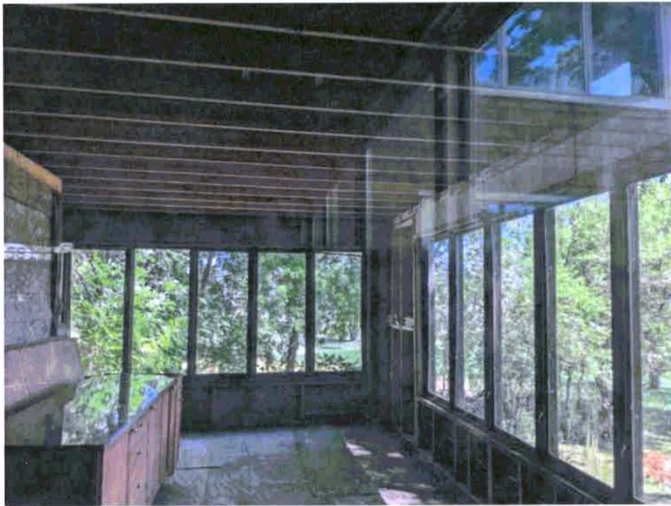
Photograph 17: Interior of second floor porch addition.
