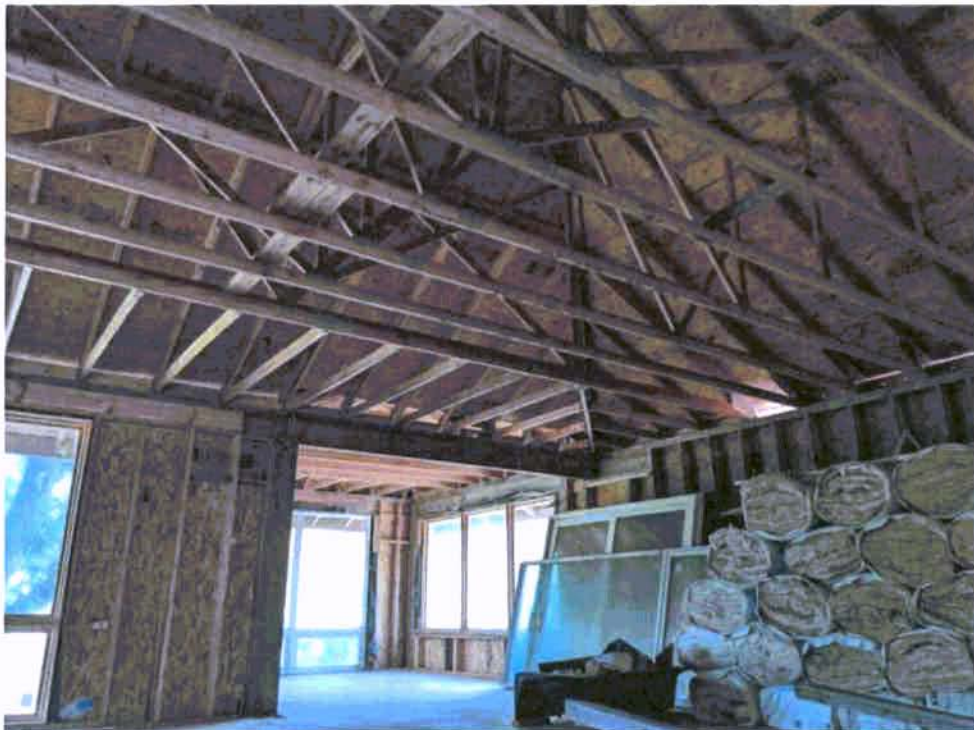
Photograph 6: Roof trusses of second floor addition (2022).
