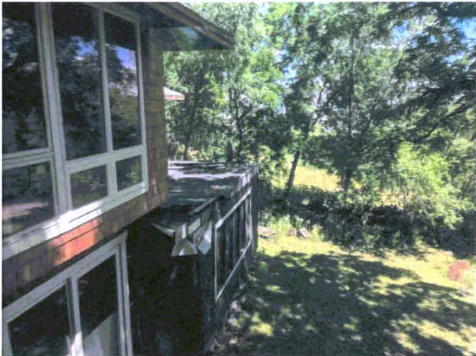
Photograph 23: Back exterior of porch.
