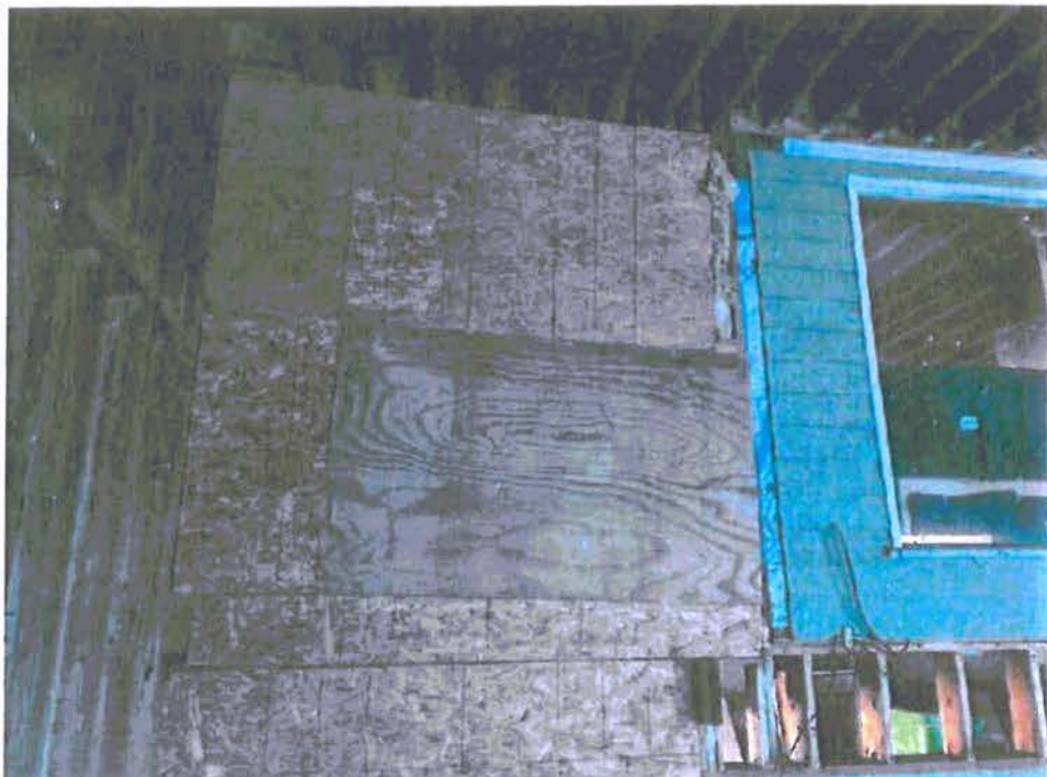
A-90: WEST WALL, SOUTH QUADRANT AT ADDITION
