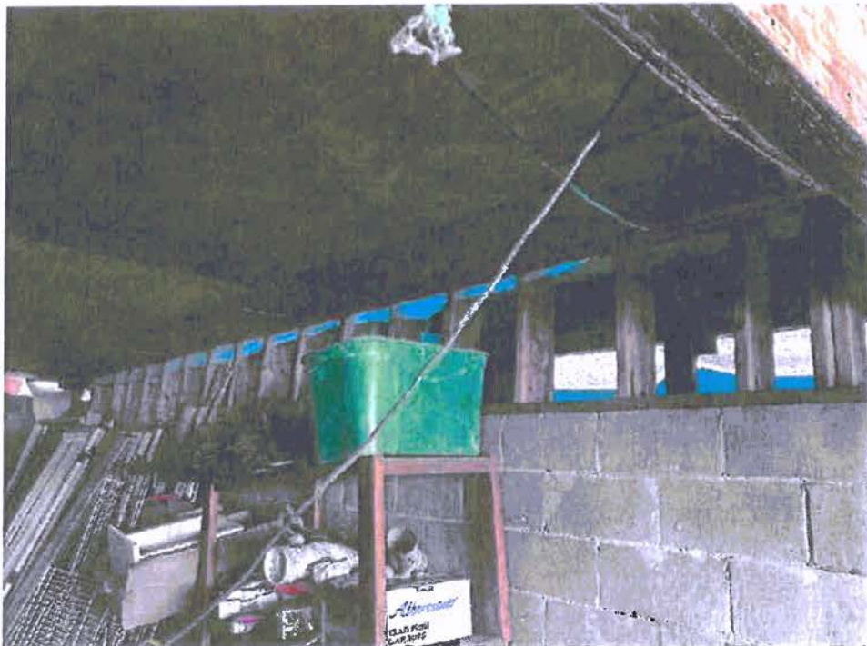
A-84: BLOCKING BETWEEN ORIGINAL EAST WALL OF HOME AND FOUNDATION WALL
