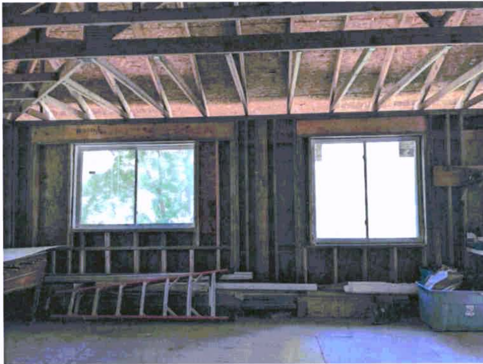
Photograph 18: Interior of second floor addition.
