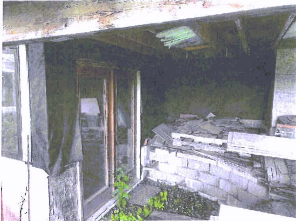
A-7: LOWER LEVEL ENTRY, EAST WALL UNDER PORCH
