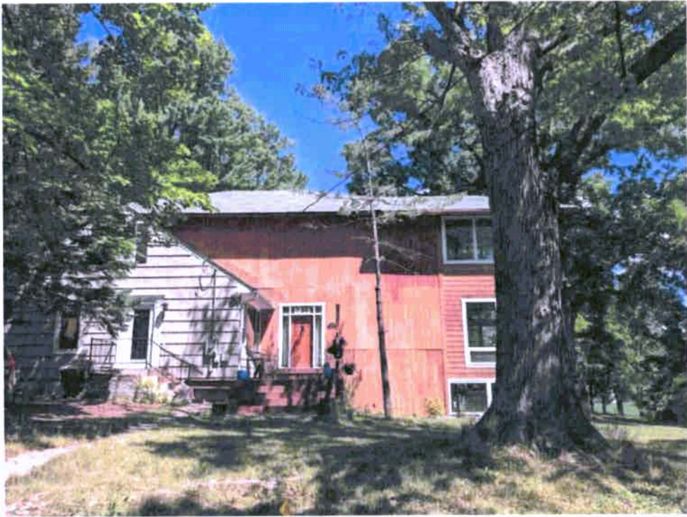
Photograph 1: Front (West) exterior of the house.
