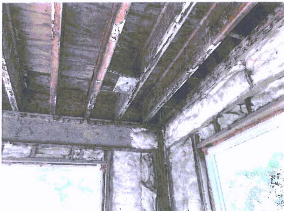
A-50: SOUTHWEST CORNER AT MAIN LEVEL
