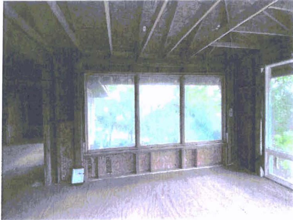
A-19: EAST WALL AT UPPER LEVEL, SOUTHWEST QUADRANT OF HOME
