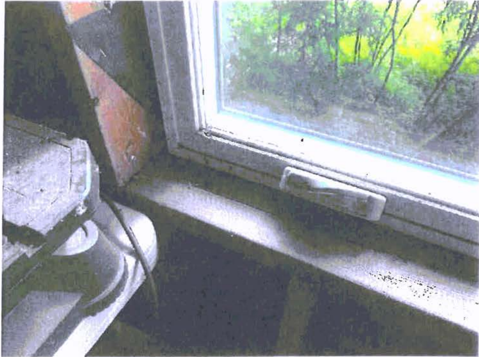
A-43: WINDOW IN EAST WALL, SOUTH QUADRANT
