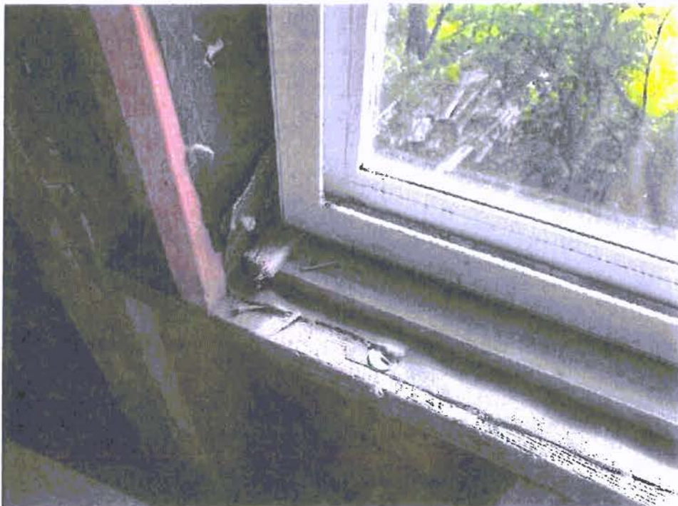
A-44: CENTER WINDOW IN EAST WALL
