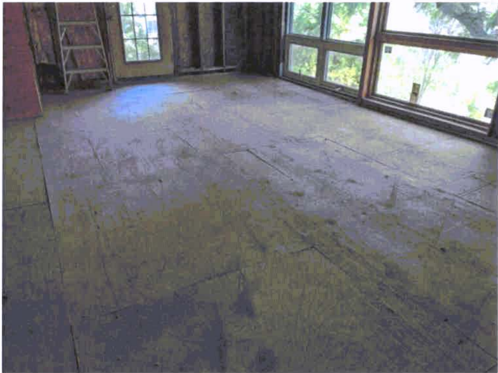
Photograph 22: Interior floor of second level addition.
