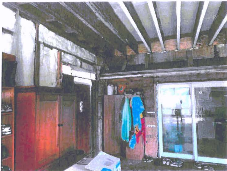
A-57: NORTHWEST CORNER OF ADDITION AT SOUTH SIDE OF ORIGINAL HOME
