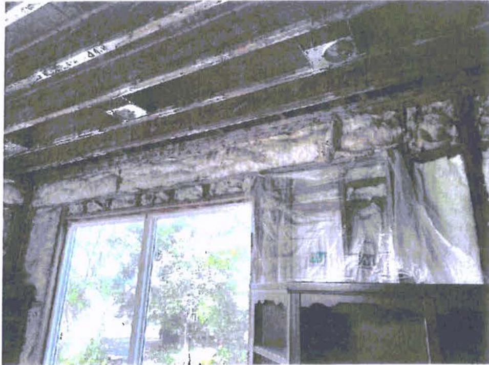
A-49: WEST WALL, SOUTHWEST QUADRANT
