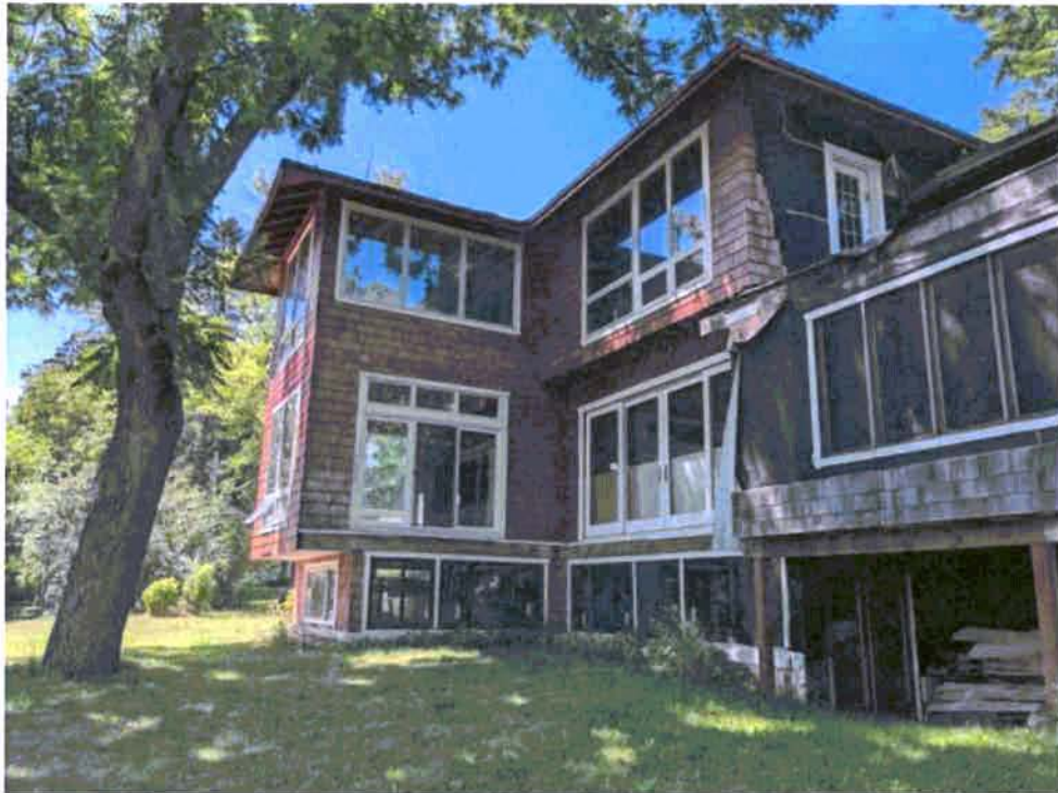
Photograph 4: South side exterior of the house.
