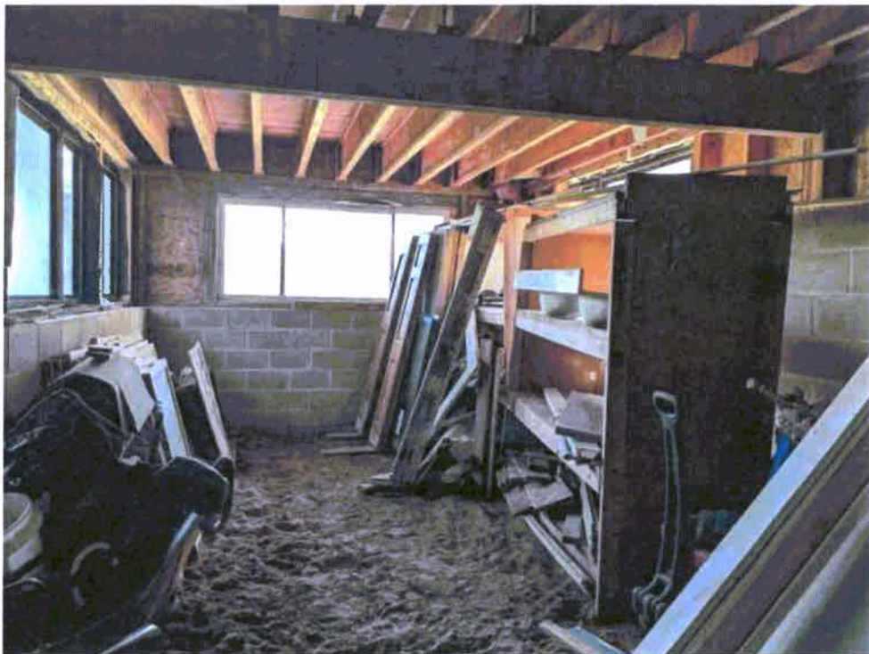
Photograph 15: Interior of basement addition.
