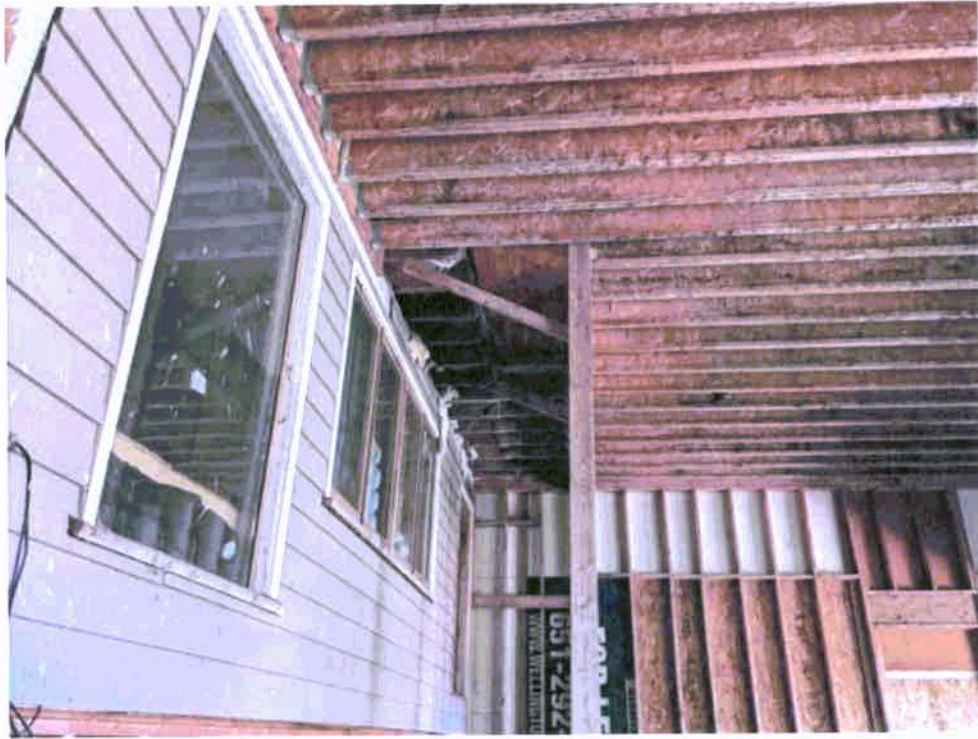
Photograph 9: Interior of garage addition.
