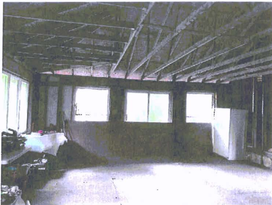
A-31: SOUTH WALL, EAST QUADRANT OF UPPER LEVEL
