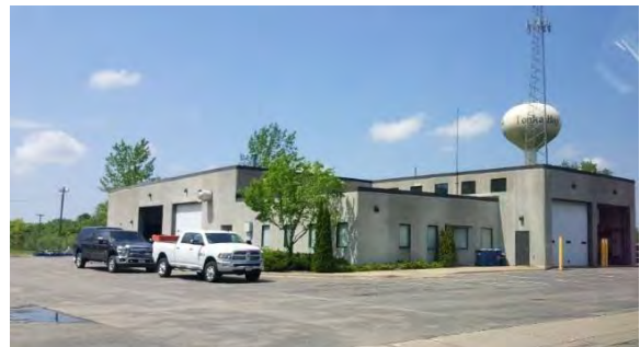
Public Works Building
