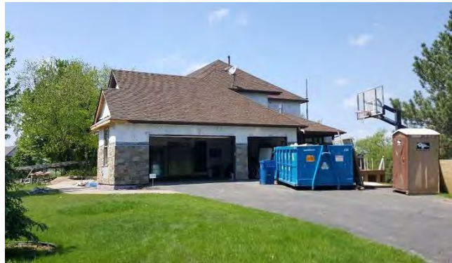
House Under Construction
