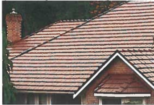
Figure 3. Metal Shingles
