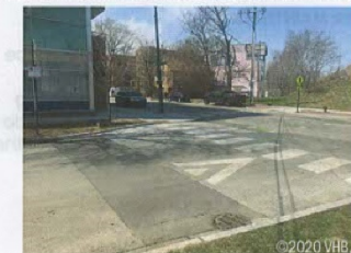
Figure 2. Photo. Raised crosswalk in Chicago with additional drainage grates added upstream of crossing.
