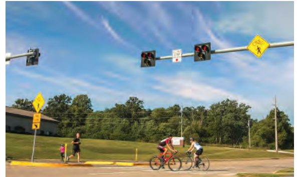
Example of a HAWK Beacon crossing
