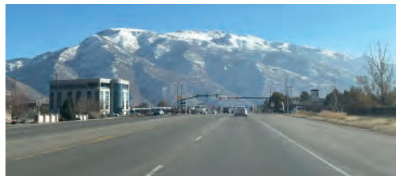
US-89, South Segment
