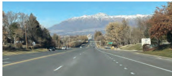
US-89, Central Segment
