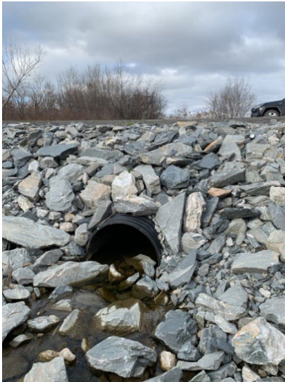
Figure 14. New cross culvert installed along Nason Street.
