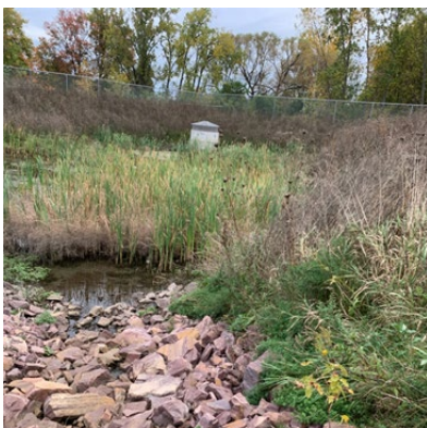
Figure 6. Gravel wetland managing stormwater from the Industrial Park and discharging to Rugg Brook.
