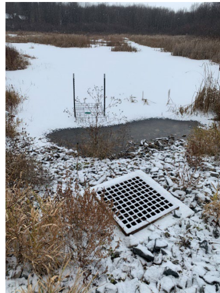
Figure 12. Inlets to the new upsized cross culvert. Note the beaver exclusion device installed.
