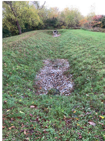
Figure 10. Dry detention pond along Loomis Lane for Thibault Meadows subdivision.
