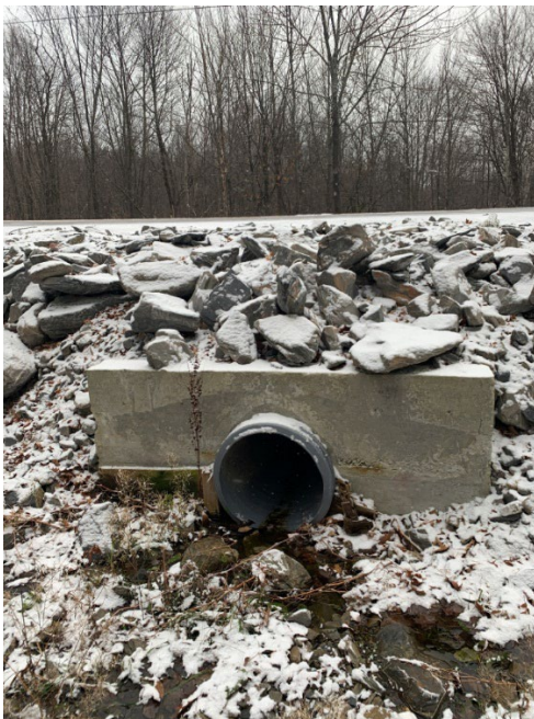
Figure 11. New cross culvert along French Hill Road.
