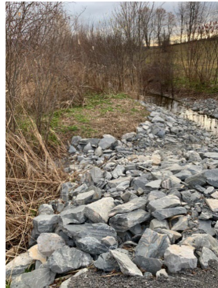
Figure 13. New stone added along ditch (south side of the road).
