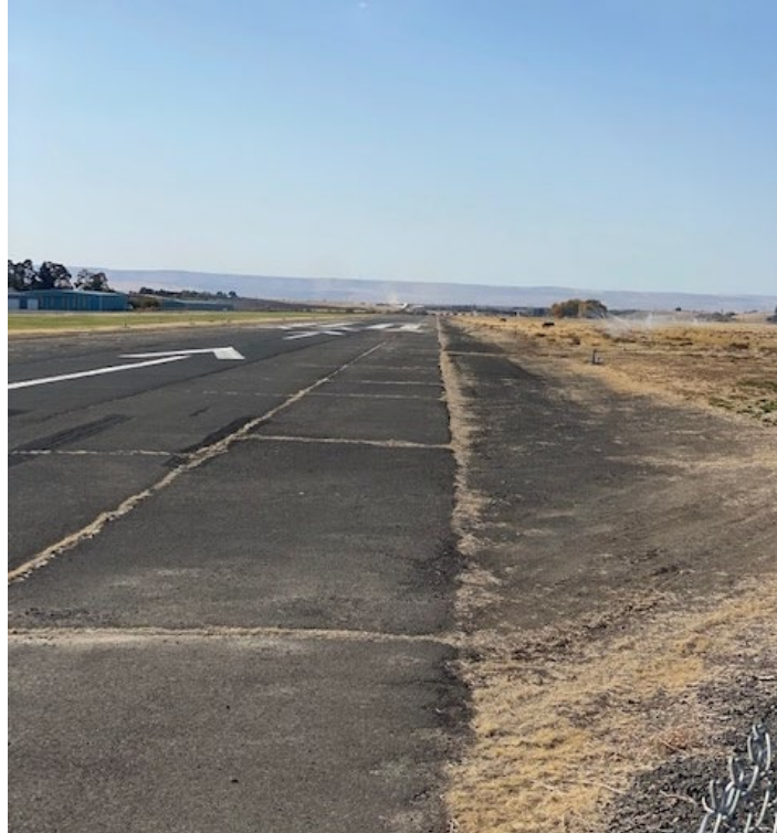
Runway shift 500 feet to the southwest. Repainted Runway approach 23 and added 500 feet to the southwest end of Runway 5.
