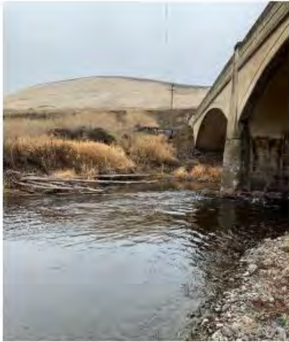
5-Looking south from the north on the upstream side of the bridge. Can see some debris upstream and protection on the embankment.
