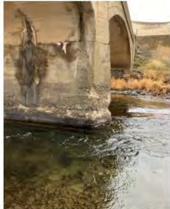
8-Looking at middle pier downstream side, also has concrete erosion and scouring. The south bank embankment on the downstream still has protection.
