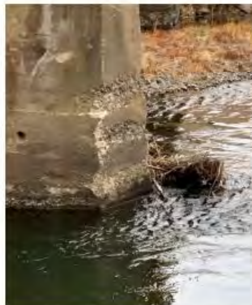
4-Closer view of the center pier that has been hit with debris and has small debris on the north side.
