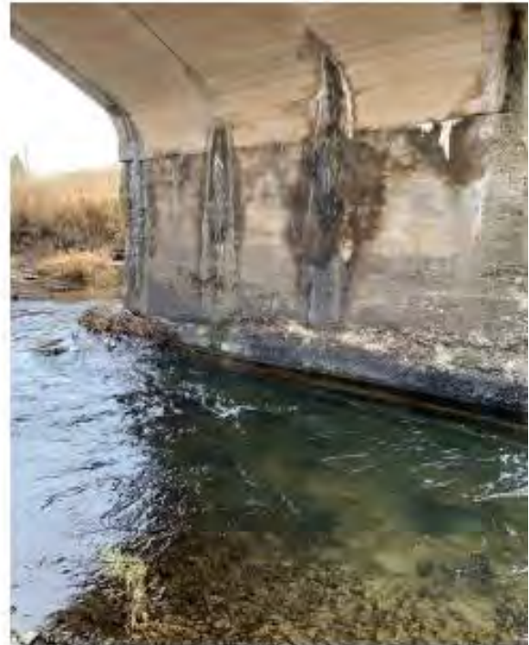
6-Looking at the center pier can see a lot of erosion of the concrete from being hit and exposed with leaching
