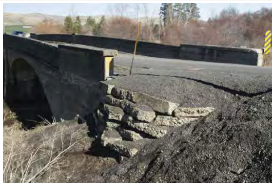
Infill Material at South Approach Looking NE.jpg
