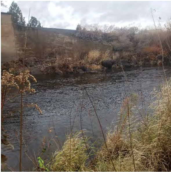
Photo 5. Bank armoring river right upstream of bridge.
