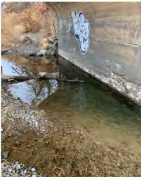
7-Looking at pier1 from upstream to downstream There is not protection left on the pier abutment and more erosion on the concrete.
