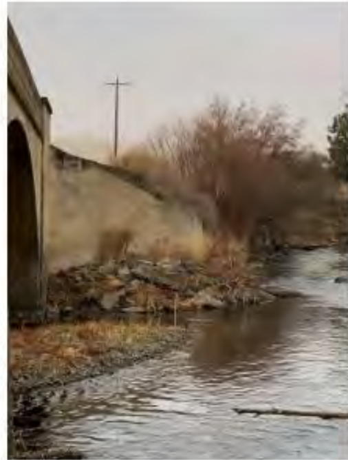
2-Looking north from the south of the bridge abutment wingwall where there is still rock protection. There's a small gravel deposition in the first span as well.
