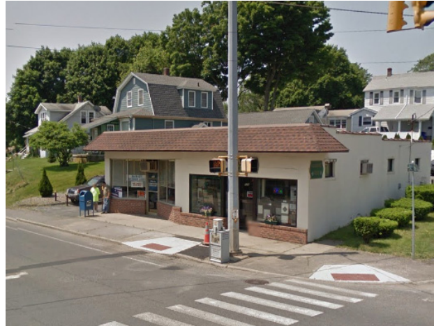
Neighborhood commercial nodes are home to small scale convenience retailers catering Watertown's village areas © Google Maps
