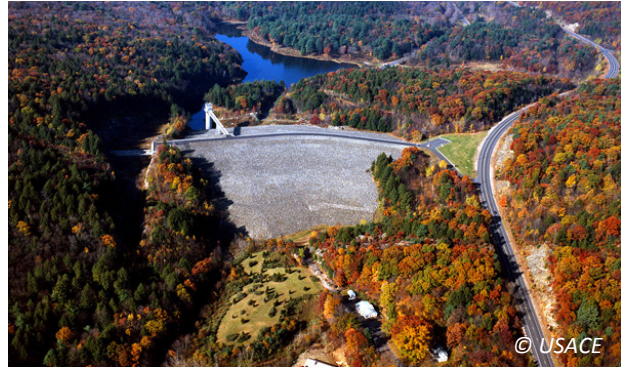
Black Rock Dam along Branch Brook is used for flood control purposes and also allows recreational activities.
