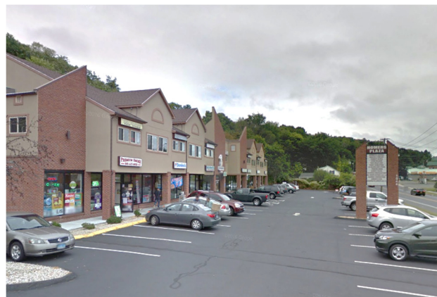
The Main Street general commercial area contains a mix of retail, office space, and services. Design guidelines could better integrate this area with Main Street in Watertown and Oakville. © Google Maps
