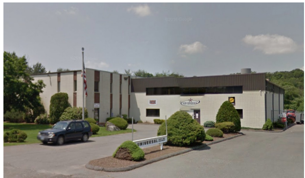
Light industrial areas are characterized by a mix of small scale manufacturing, distribution, and wholesalers. © Google Maps
