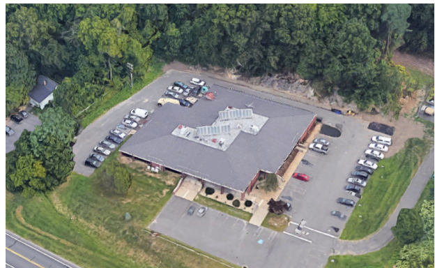
The Watertown Police Department Headquarters was built in 1980 and meets the operational needs of the department.
