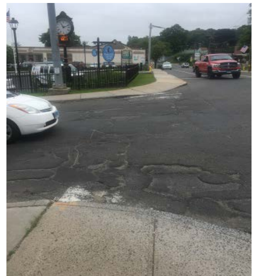
Figure 15. Faded crosswalk, poorly located pedestrian push button
