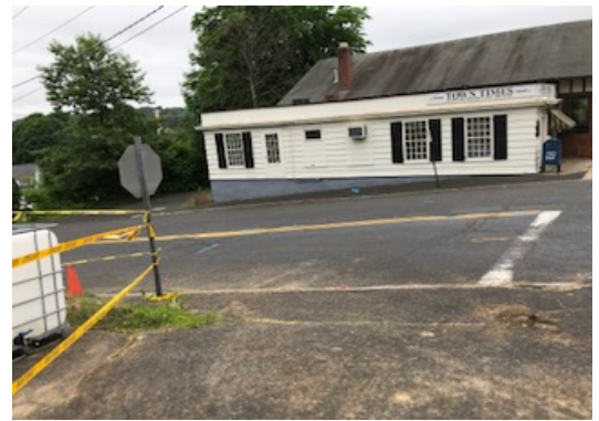
Figure 13. Stop bar and stop sign not aligned
