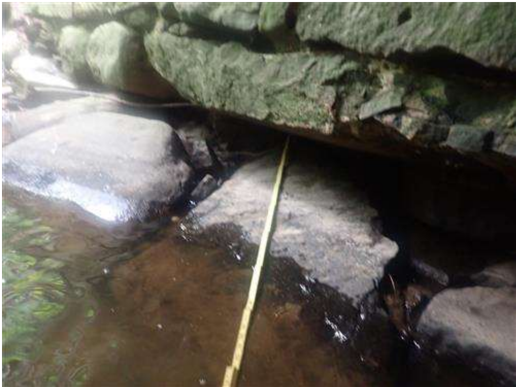
Stick ruler measuring the depth of void near the inlet end of abutment # 2.
