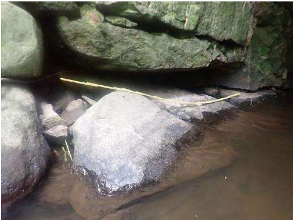
Six foot the length of large void at the base of abutment # 2 near the inlet end.
