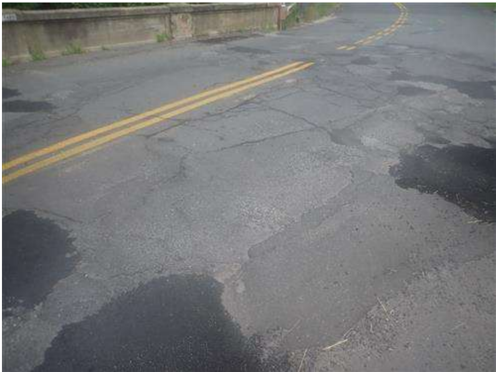
A closer view of the bituminous concrete wearing surface.
