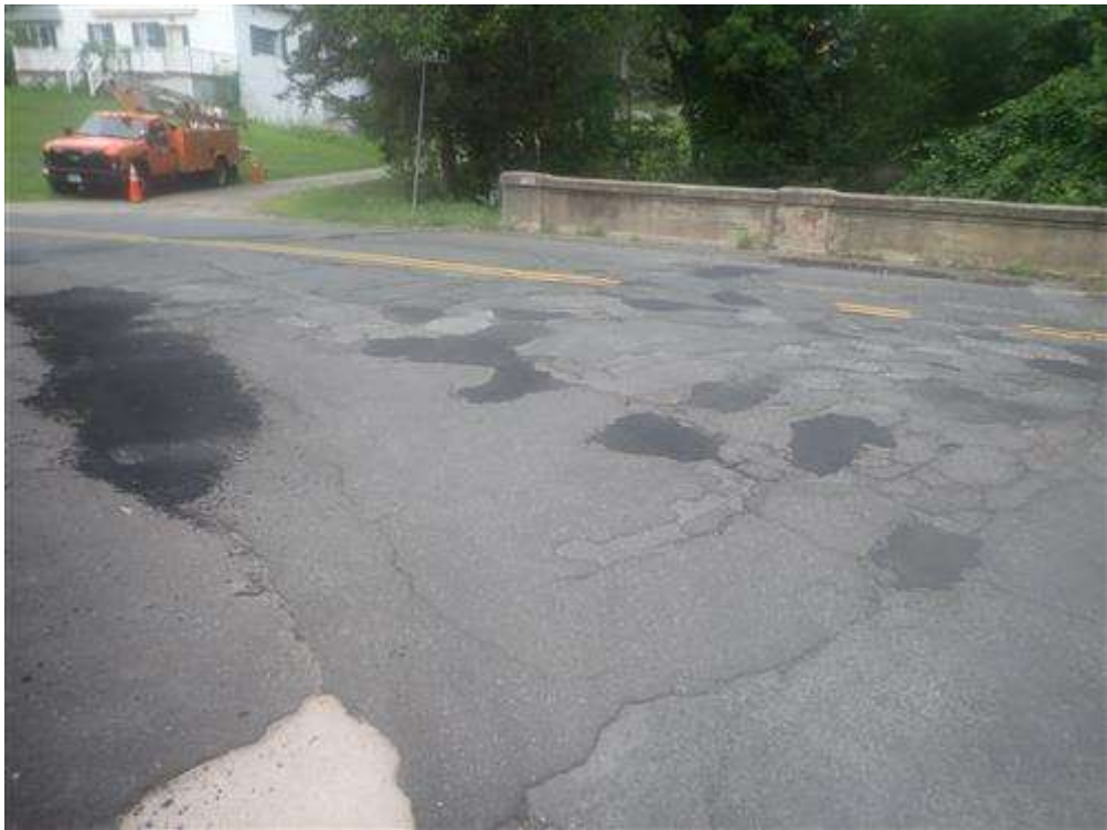
General bituminous concrete wearing surface with numerous patches and cracks.
