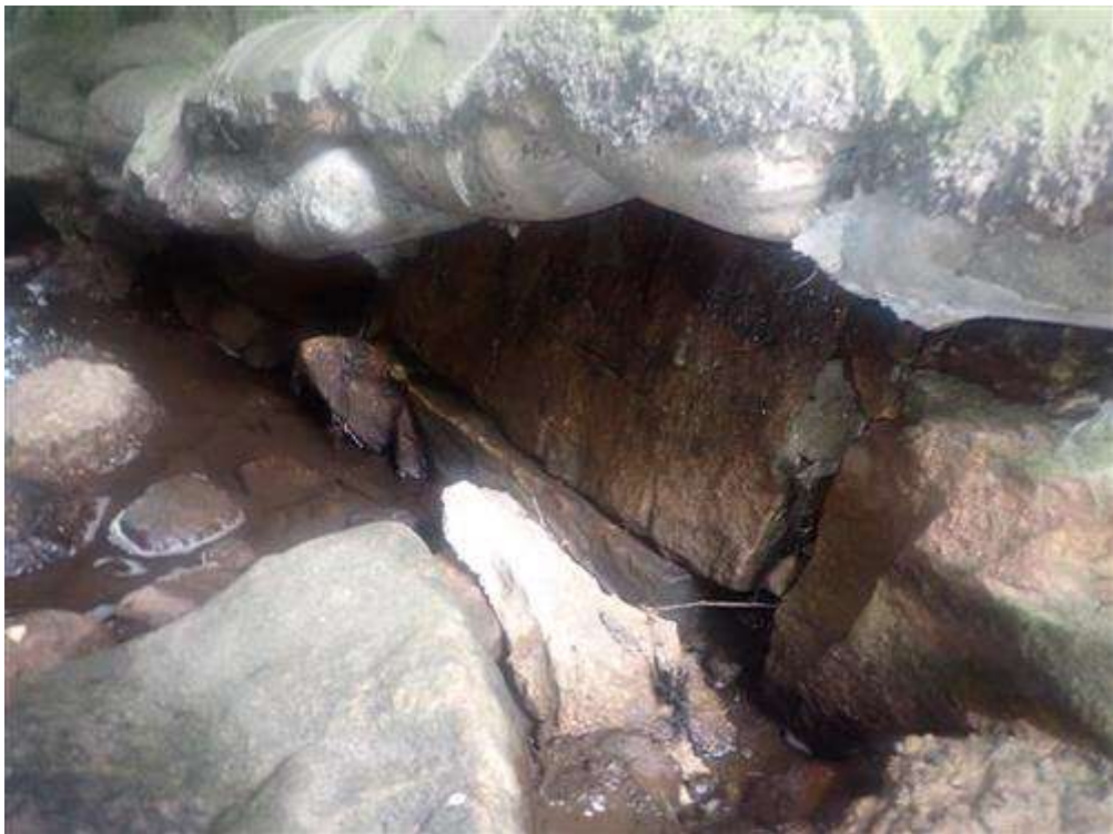
Void at the base of abutment # 1 near the inlet end.
