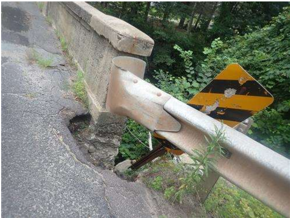
View of the undermining of roadway at the Northwest corner.
