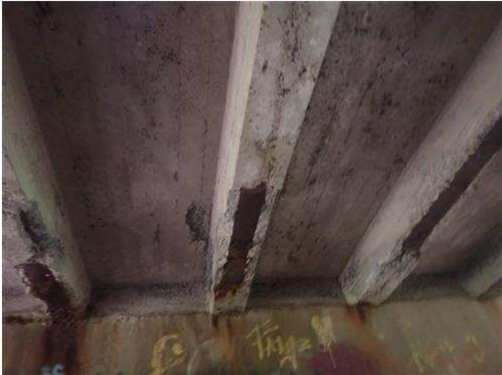
Typical missing concrete at the bottom flange's of beams in span # 2.
