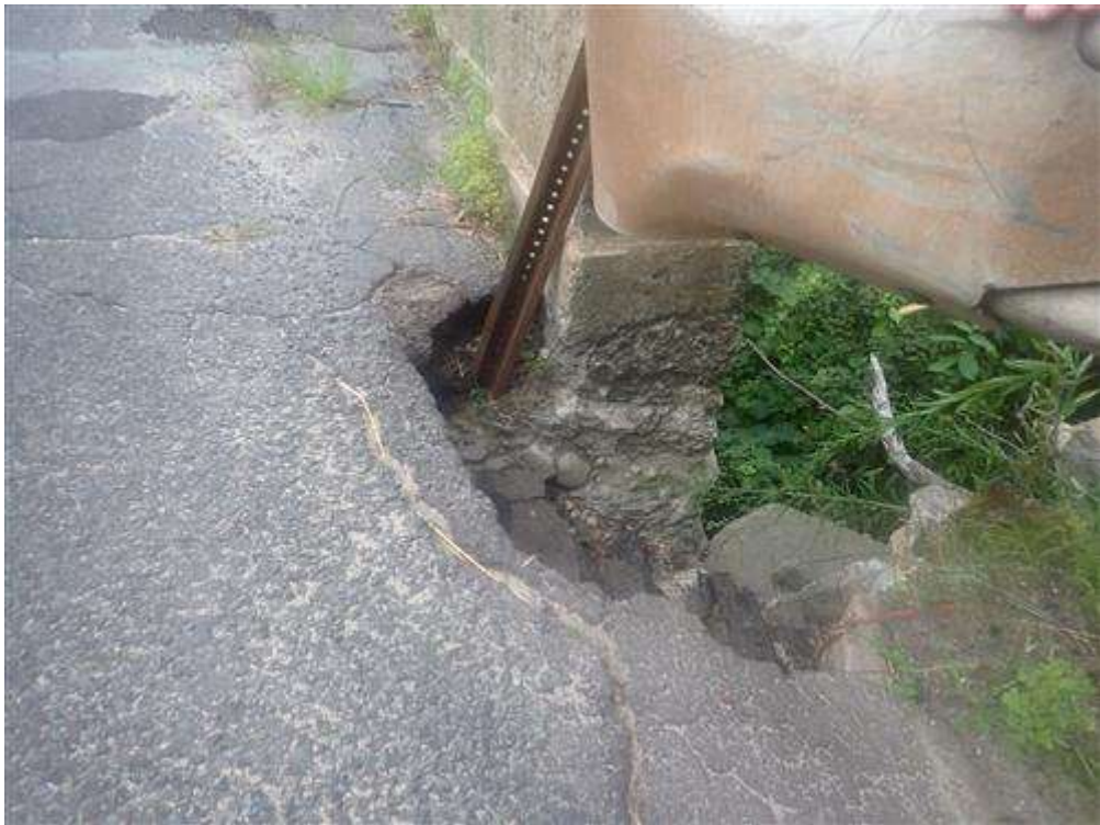
A closer view of the undermining of roadway at the Northwest corner.
