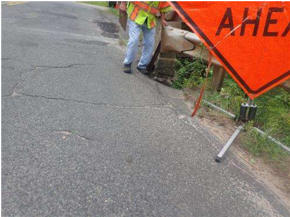
Lead inspector investigating undermining of Bituminous concrete at the Northwest corner of structure.
