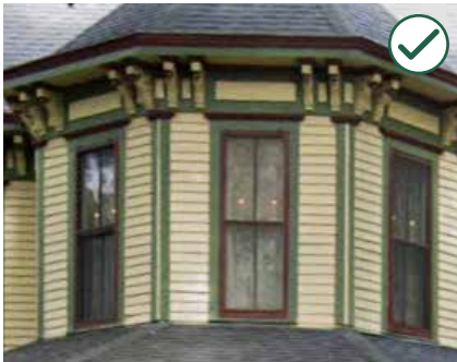
Preserve the position, number, size and arrangement of historic windows on a building wall.
