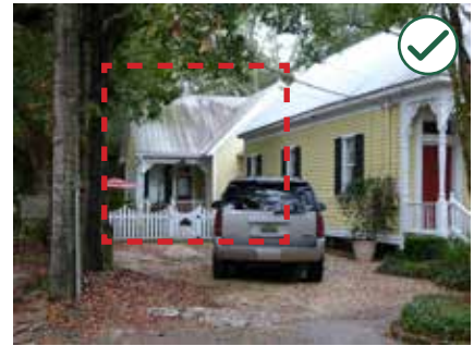
Use simplified versions of building components and details found in the historic context.
