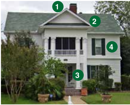
520 North College Street, an example of Classical Revival architecture.
