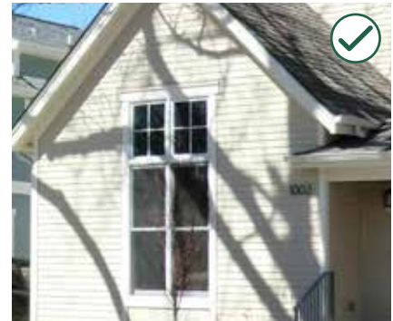
Create a solid-to-void ratio similar to that seen on nearby historic buildings.
