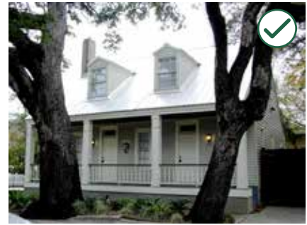
A metal roof with a low profile standing seam is an acceptable roof replacement material.
