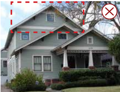
Scale a rooftop addition to ensure the historic structure remains visually prominent. This addition overwhelms the original building.
