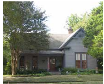
Three photos taken over the 100+ year history of 817 W. Main show how key character-defining features were preserved during the most recent improvements to the exterior of the structure.
