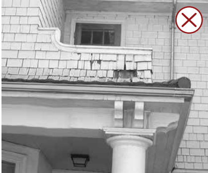
Repair a deteriorated primary building material.
