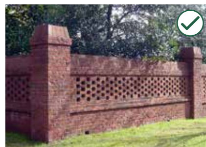
Preserve historic fences, gates and walls.
