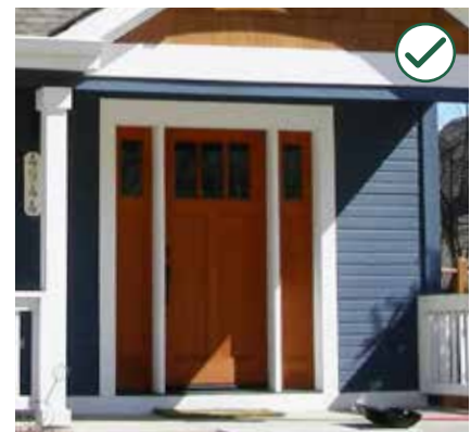
Materials that are the same as the original, or that appear similar in texture and finish to the original, such as the wood door with glass lights above, are acceptable.
