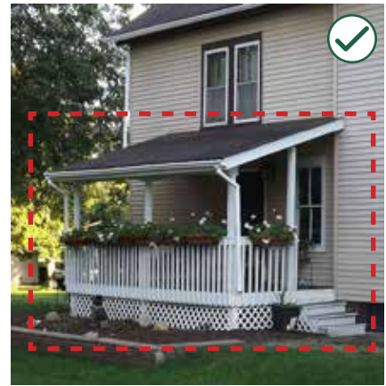
Design the scale and proportion of a porch addition to be subordinate to the existing historic residential structure.
