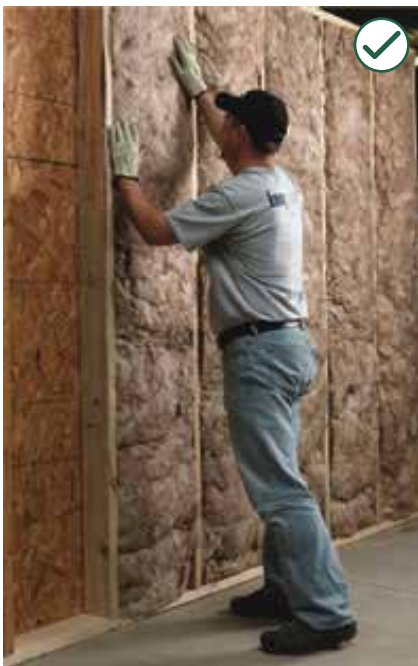
Use noninvasive strategies when applying weatherization improvements. This insulation is being placed on the interior wall.
