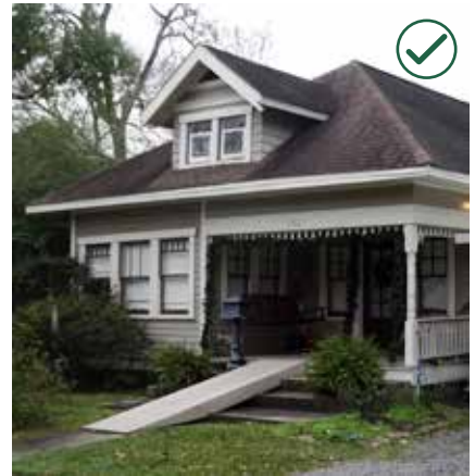
Create an accessibility solution that can be reversed. For instance, a ramp could be installed and then removed without affecting the historic building.
