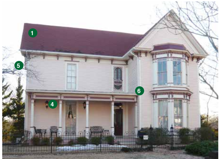
417 West Jefferson Street, a contributing structure in the West End Historic District and an example of the Queen Anne style.
