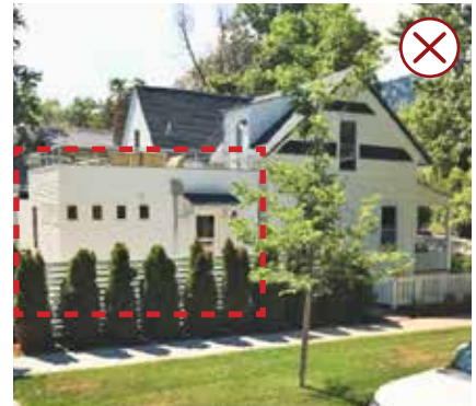
Where an addition is visible from the street, design it to respect the solid-to-void ratio of, and to preserve the rhythm of doors and windows on, the historic building.
