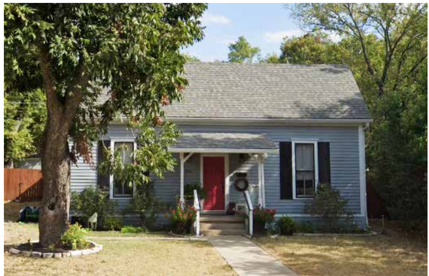
104 Bryson Street, an example of the National Folk style that utilizes the hall-and-parlor layout.
