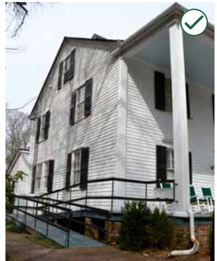
Locate an access ramp to the side or rear of a building.
