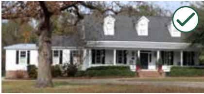
An addition constructed in a manner compatible with the original building and associated with the period of significance may merit preservation in its own right.
