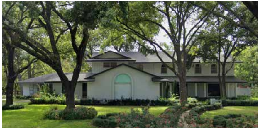
801 West Main, an example of the Post-Modern style.
