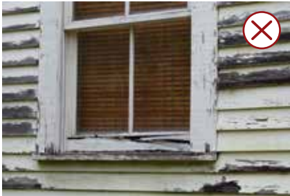
Repair frames and sashes rather than replacing them, whenever possible.
