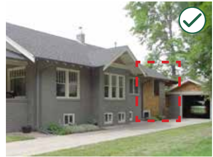
Design an addition to be generally compatible with, but distinguishable from, the historic building.
