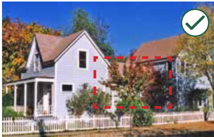
Consider using a lower-scale connecting element to separate an addition from the historic structure.
