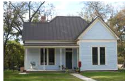
The Residential Design Guidelines provide guidance for rehabilitation projects to ensure appropriate alterations are made. The images above illustrate one such project, with the top photo showing 1009 W. Main before rehabilitation, and the bottom image taken after the project was completed.
