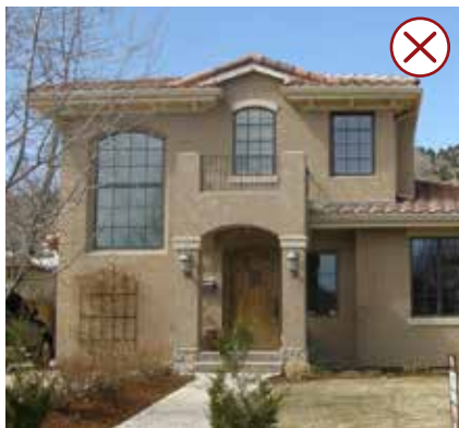
This building is not compatible with Waxahachie’s residential historic districts. Its windows and entry features are out of proportion with others in the context.
