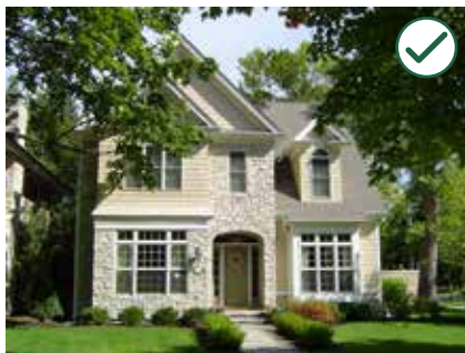
Design a dormer to be in scale with the roof and with those used traditionally in the neighborhood. This dormer is appropriate where the historic context includes front-facing dormers.
