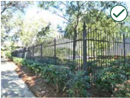
Materials that have a similar character, durability and finish to those of fences of historic properties, such as the iron fence seen above, are acceptable.
