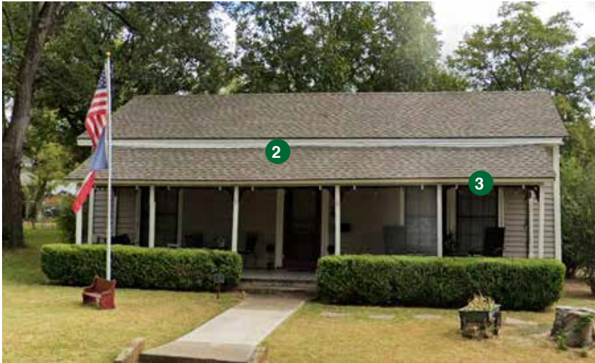
209 South Hawkins Street, a contributing structure to the West End Historic District and an example of the Folk Victorian style.
