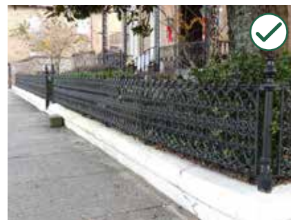
Maintain any distinctive details and protective finishes.
