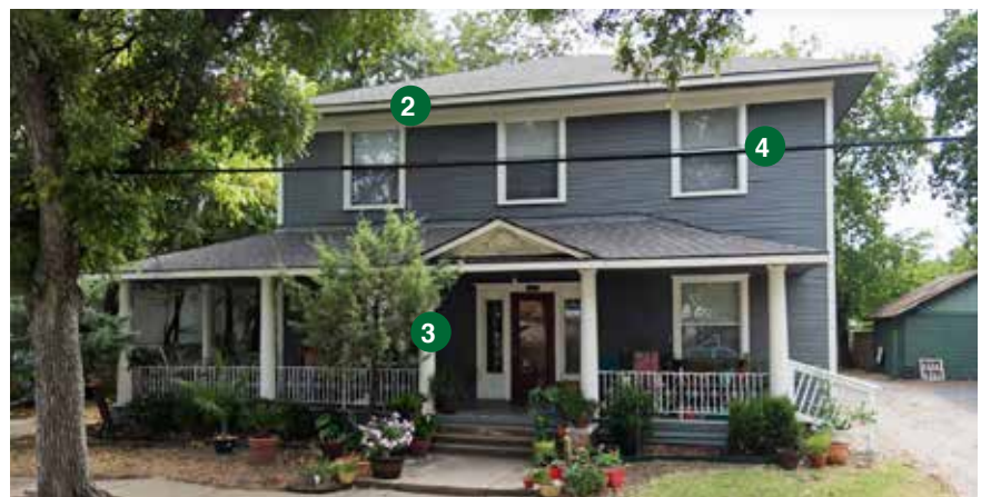
409 West Franklin Street, a contributing structure to the West End Historic District and an example of Classical Revival architecture.
