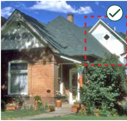
Design a roof of an addition to be compatible with, but visually subordinate to, the existing historic building.
