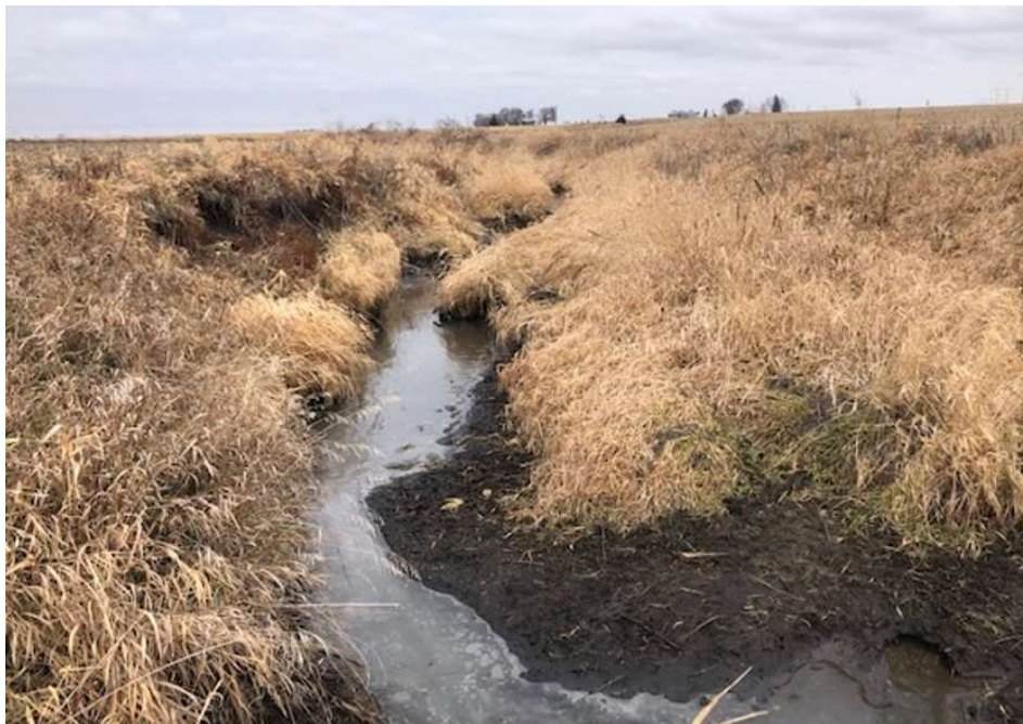
Image 2: Example of meandering and silt accumulation. The sideslope on the right side of the image has sloughed into the ditch and caused the creek to meander and erode the bank on the left side.
