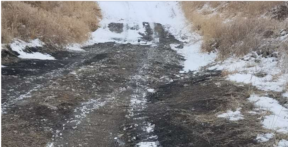
Image 4: Low water crossing of rock and soil
