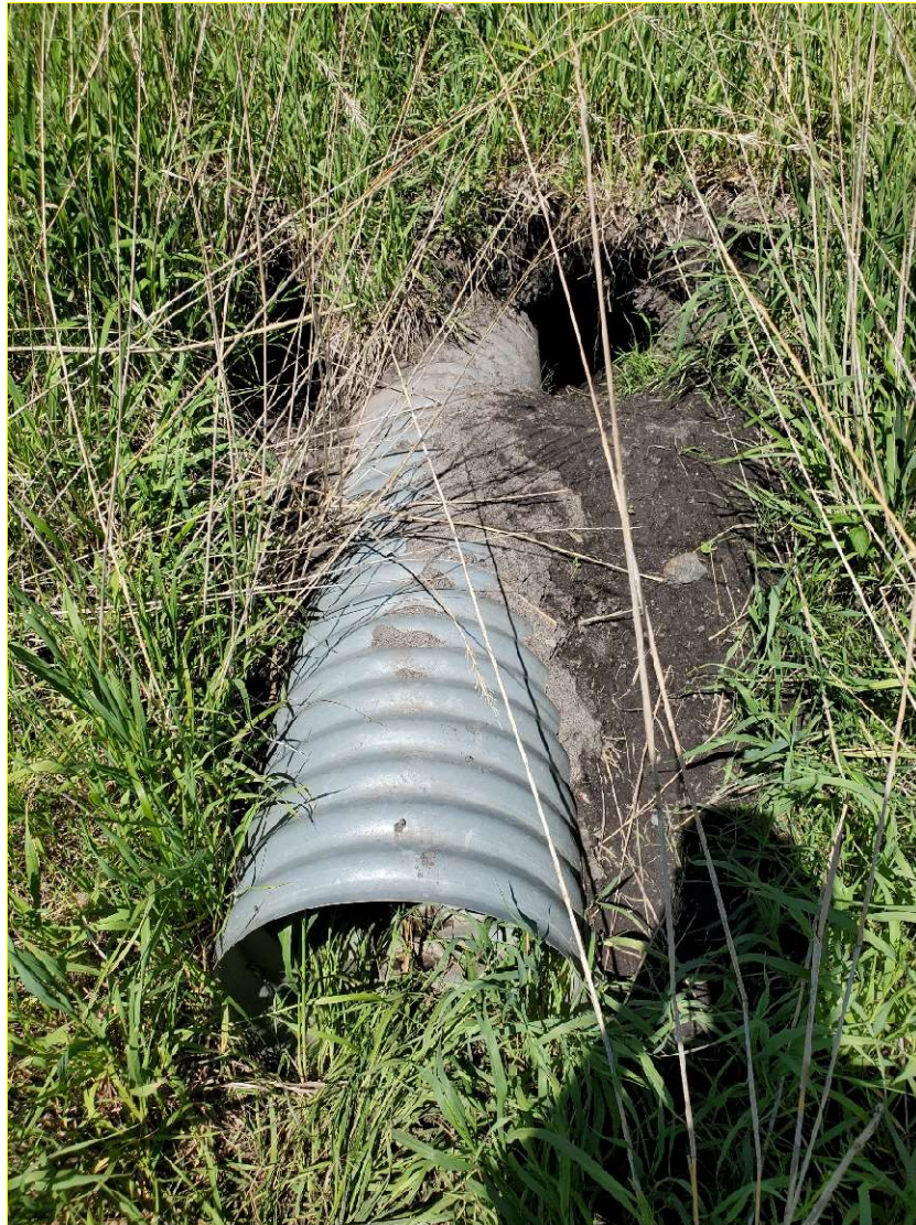
Image 5: Pipe with bypass erosion
