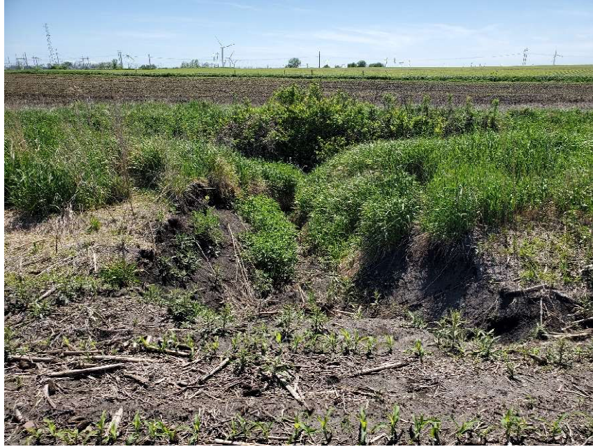
Image 1: Example erosion caused by surface water eroding from above the ditch bank. This failure is commonly referred to as a head cut.
