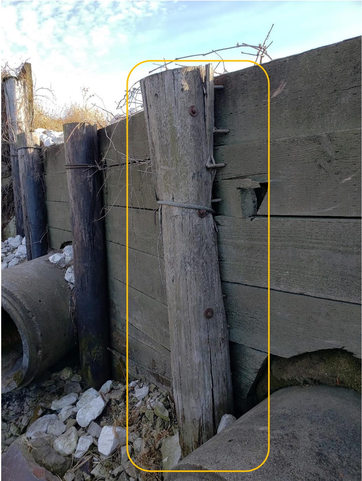
Figure 3: Another view of the broken pile and adjacent broken cross member
