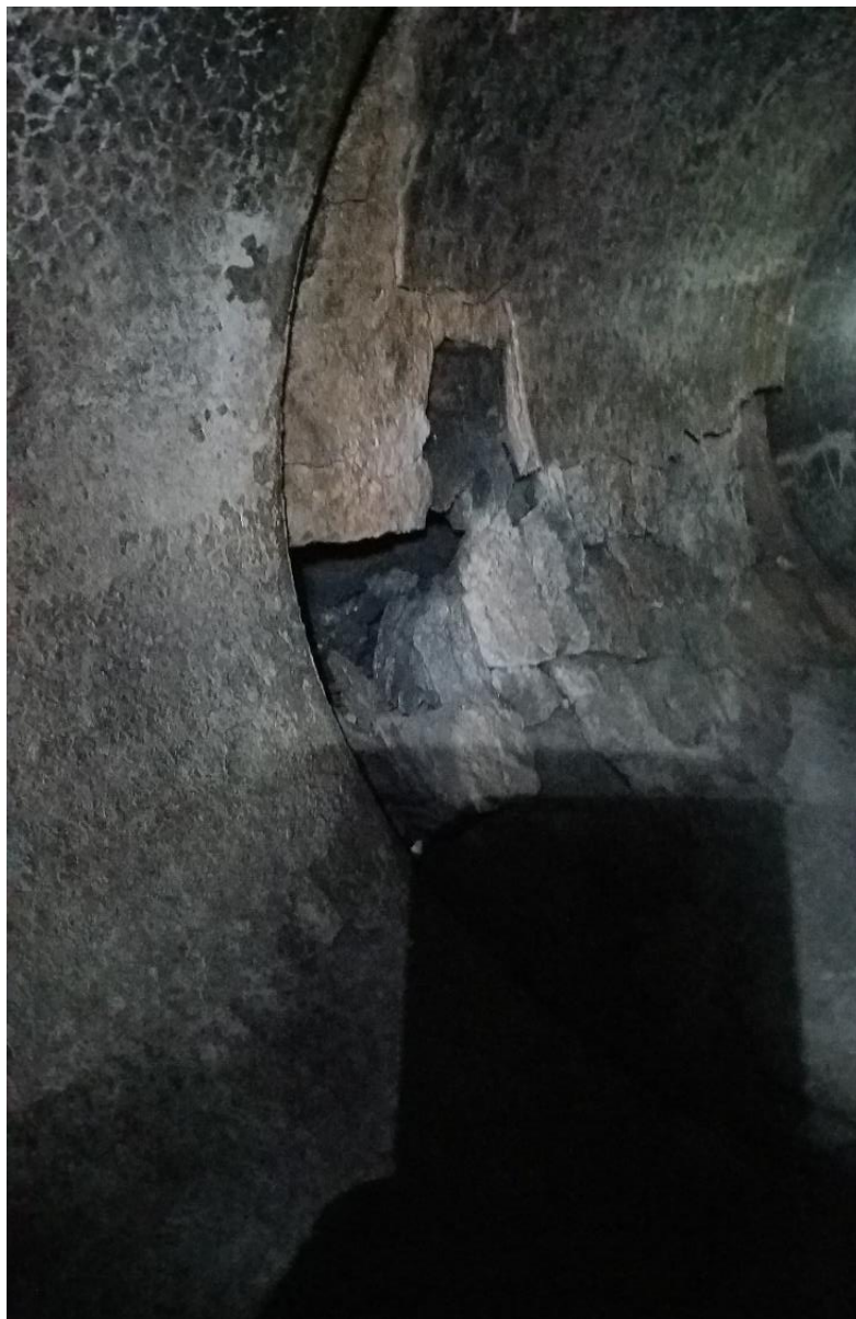
Figure 6: Lateral A broken 30" clay pipe segments.
