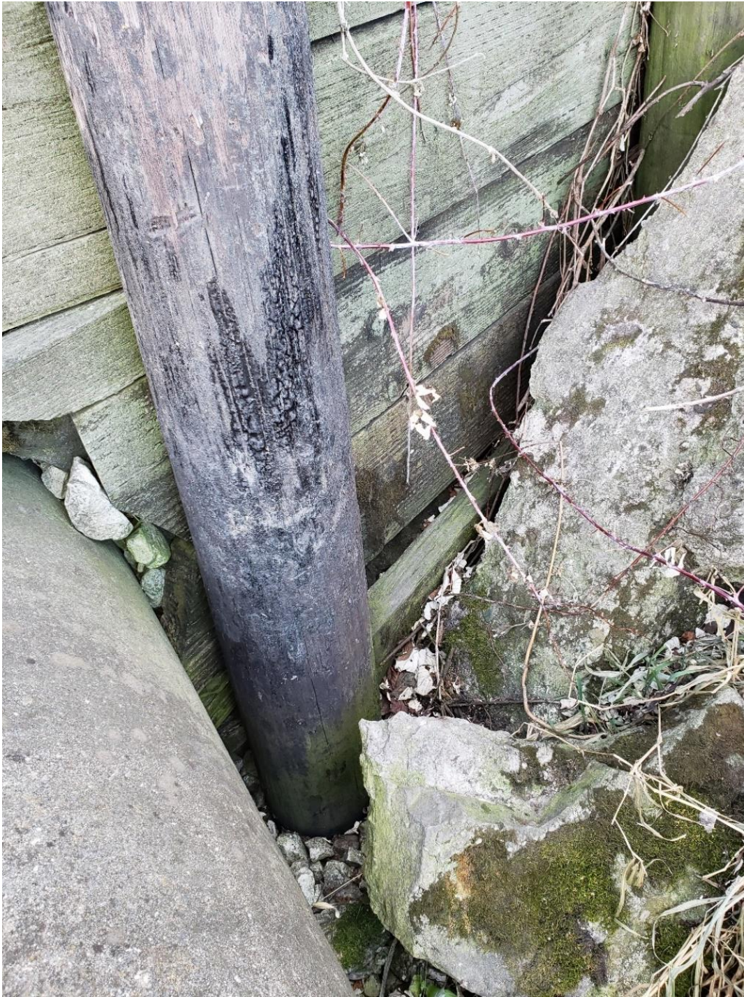
Figure 5: Base board failing.
