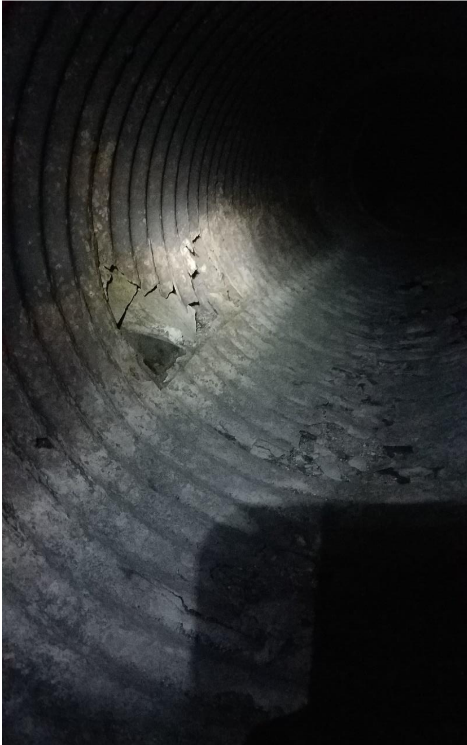
Figure 7: Lateral A deteriorating 30" CMP.
