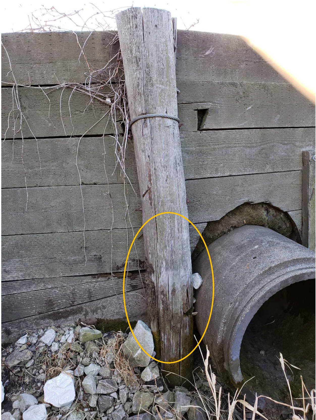
Figure 2: Broken pile allowing buckling next to Lateral C
