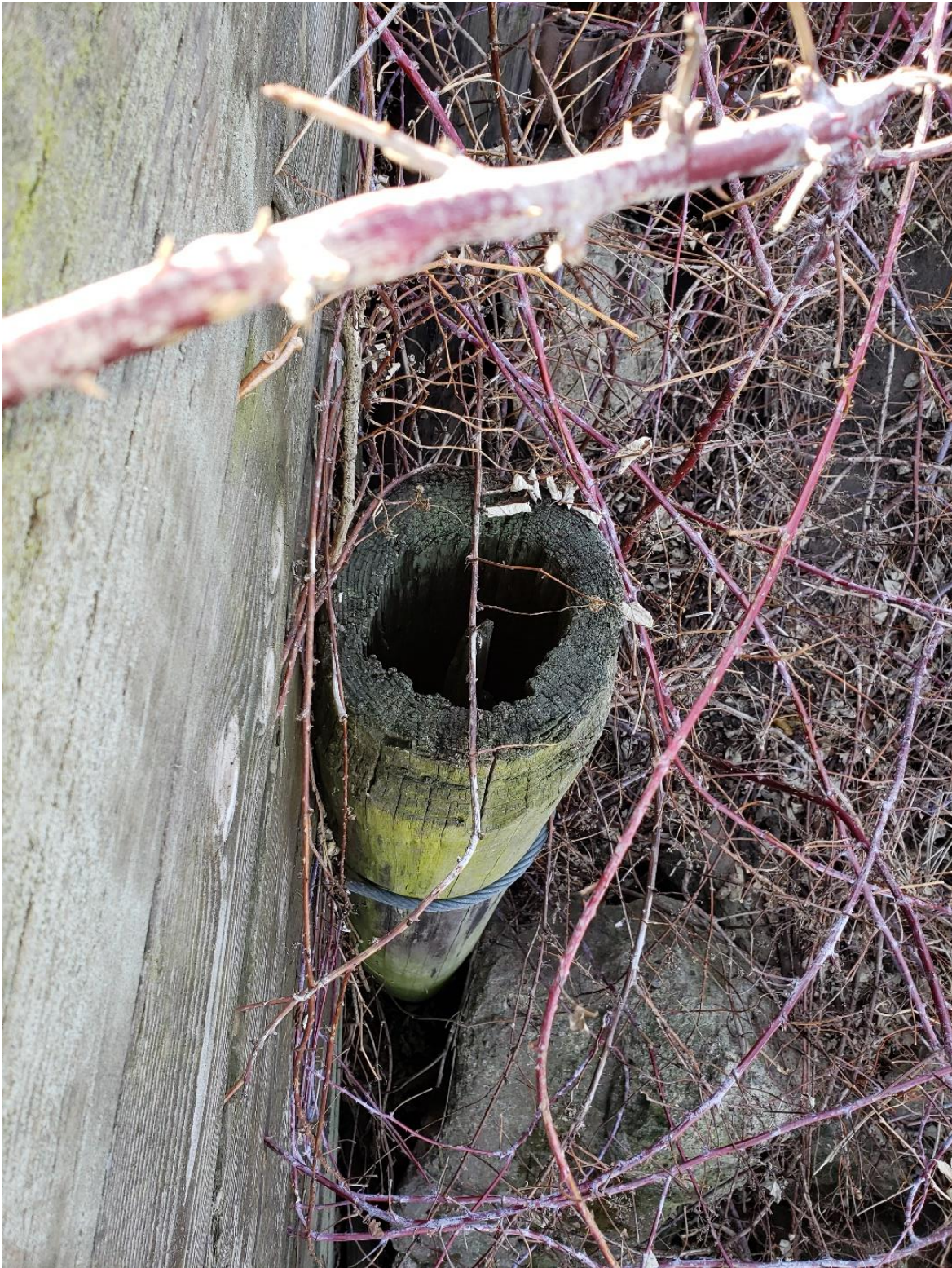
Figure 4: Another pile experiencing deterioration on the top, center.
