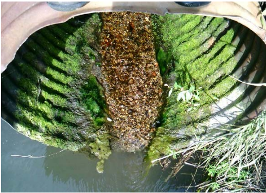
Figure 5: Silt in outlets
