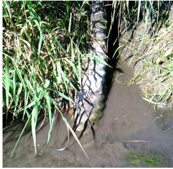
Figure 4: Outlet submerged in silt
