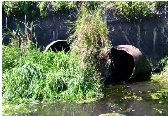
Figure 6: Erosion around headwall
