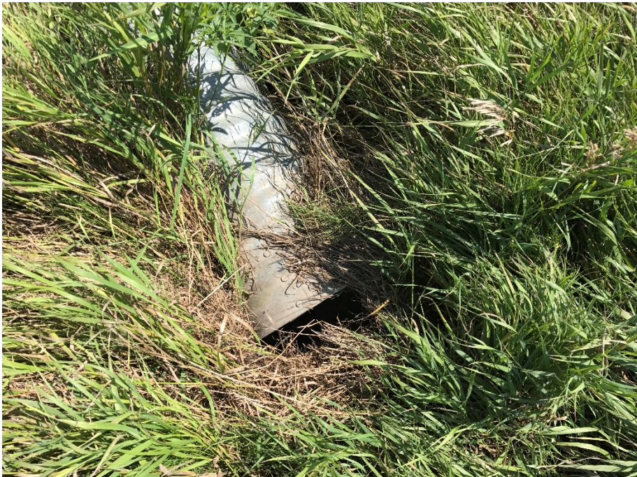
Figure 1: Submerged and sinking outlet
