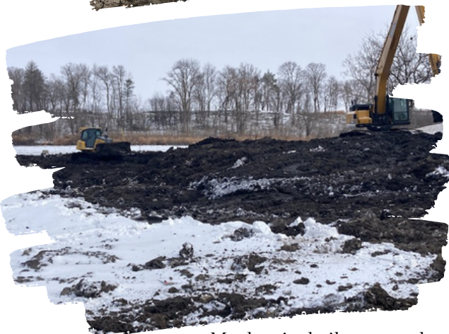
Mechanical silt removal
