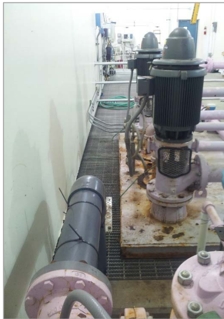
Photograph 5-3. Corrosion Damage on Reclaimed Water Pump Station Pump Skid
