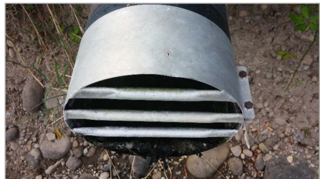
Photograph 5-5. Centralia Power Canal Outfall Pipe Screen
