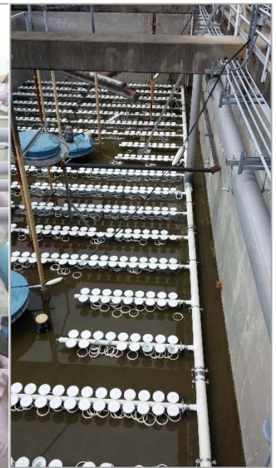
Photograph 5-4. Single Aeration Diffuser Grid in Deep SBR Tank
