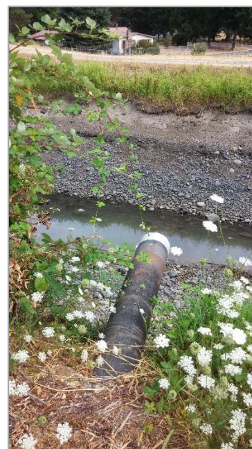
Photograph 5-1. Outfall Pipe to Centralia Power Canal
