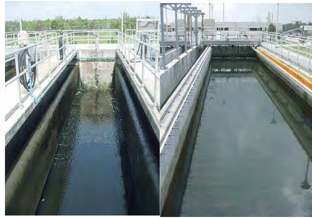
Figures 1 and 2. Denitrifying filters at the East Central Regional Water Reclamation Facility, West Palm Beach, Florida
