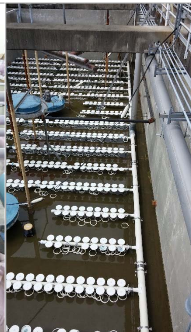
Photograph ES-7. Single Aeration Diffuser Grid in Deep SBR Tank
