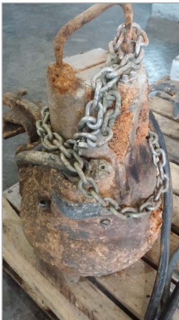
Photograph ES-5. Worn Reject Water Pump Station Pump
