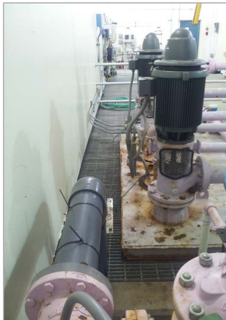
Photograph ES-6. Corrosion Damage on Reclaimed Water Pump Station Pump Skid
