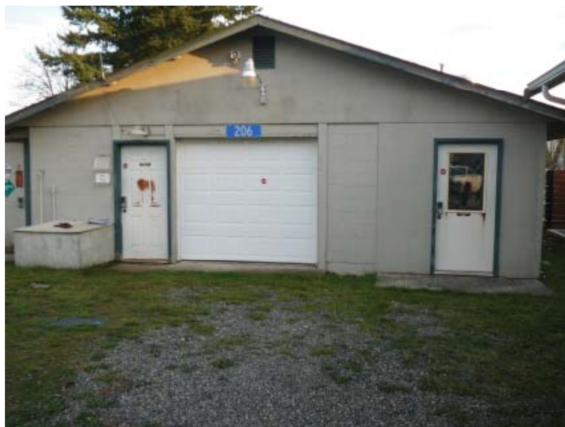
Figure 4: Well #1 Pumphouse/Storage Building
