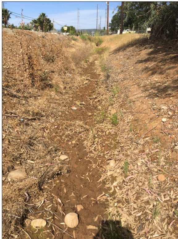
Photograph 12: West of Photograph 11, view of roadside ditch RD-7, which contained flow lines and sediment sorting.
