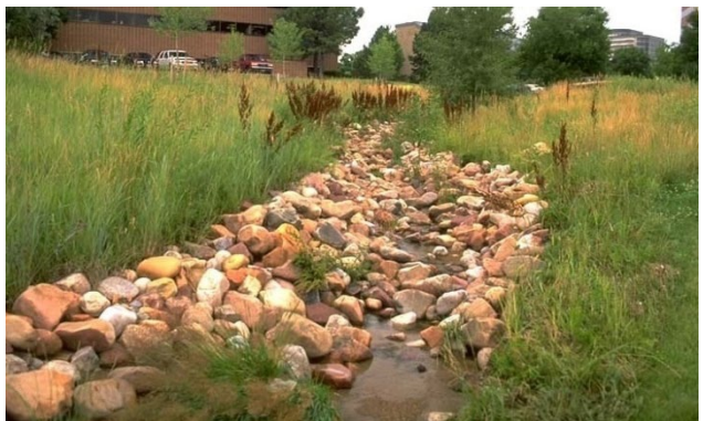
Top Photo: Vegetated areas can be used in parking lots to slow stormwater and promote groundwater infiltration.
