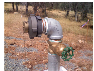
Example of hydrant and fittings
