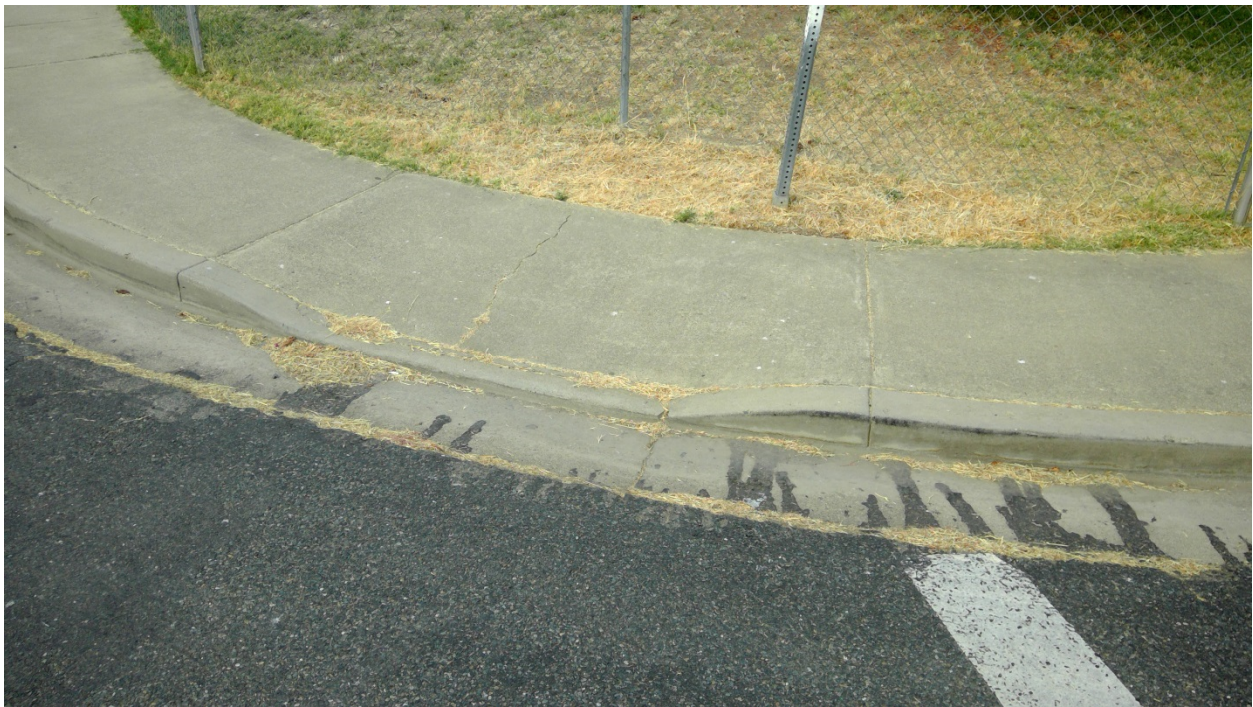
Figure 5: Example of ADA non-compliant curb ramp (Data entry #181)
