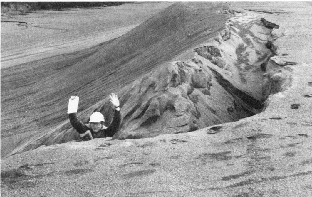
**Figure 5-5. Routine dam inspection is a necessary part of a dam safety program. This rather dramatic erosion problem was identified during a routine inspection. Source: Minnesota Dept. of Natural Resources.**
