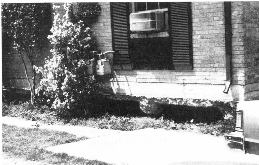
**Figure 9-3. Subsidence on organic soils has resulted in structural damage to this house in New Orleans. Source: B. Cox.**
