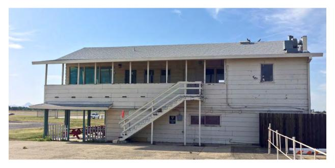
**Figure 4.** This airport building is in need of paint and maintenance. Airport buildings do not have scheduled maintenance and are now showing signs of wear. The exposed wood and leaking roofs are beginning to require funding and maintenance. Aircraft and equipment are reportedly getting wet in these facilities because of leaking roofs.
