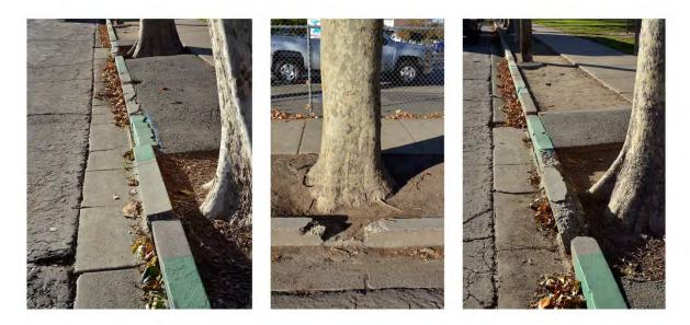
**Figure 3.** Broken Curbs on the part of 7<sup>th</sup> Street that traverses the Covillaud Elementary campus.
